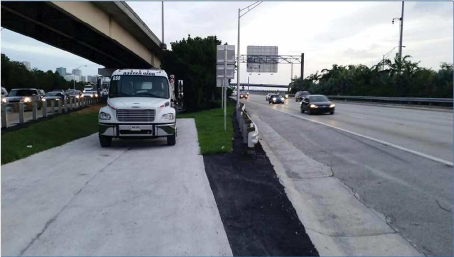
Staging area for incident management.
