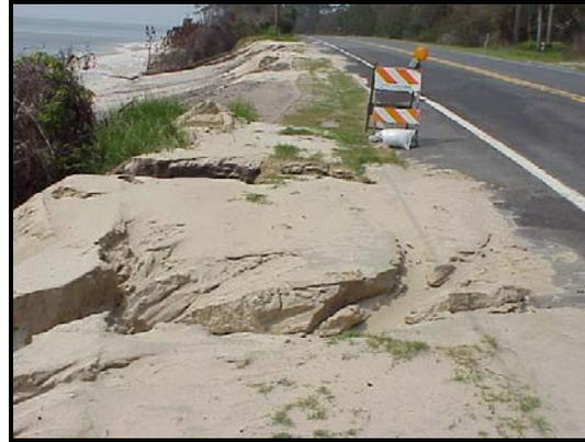
*Sheet and gully erosion along shoulder, August 2005*
