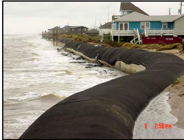
*Sandsock, sand-filled tubular geotextile
