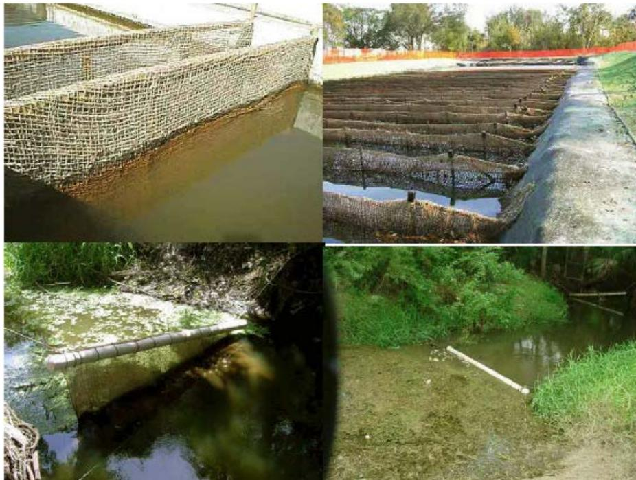
Figure AIII-25: Polymer-enhanced Particle Curtains.
