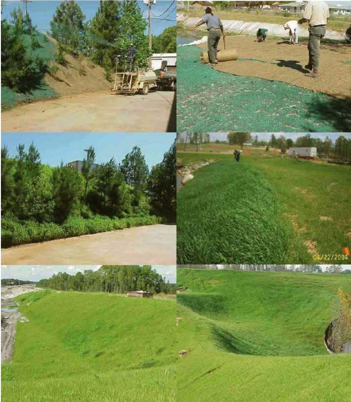
Figure AIII-7: Polymer-enhanced Turf Reinforced Matting.
