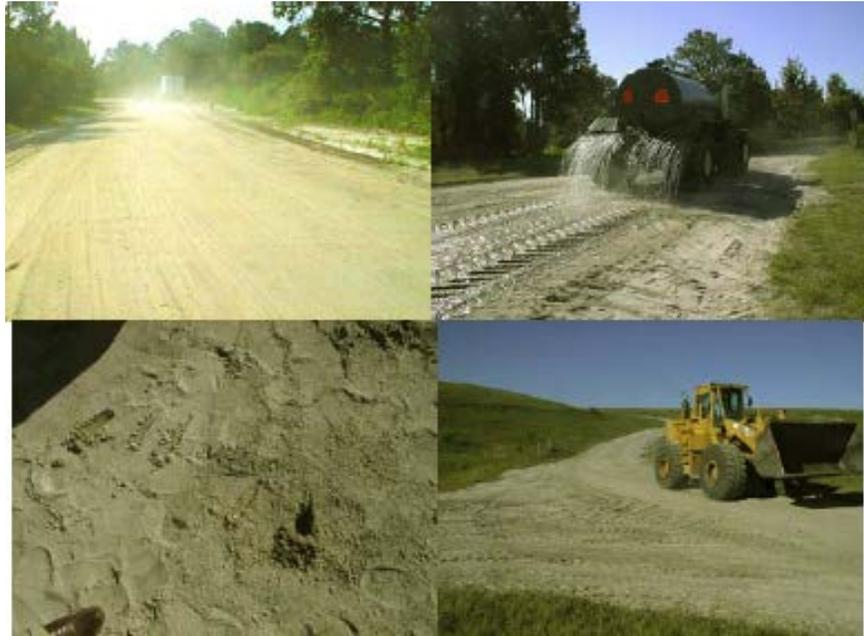
Figure AIII-29: Polymer-enhanced Dust Suppression.
