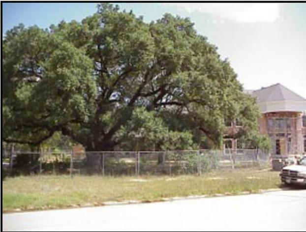
*Protected tree on construction site, with fencing outside dripline
