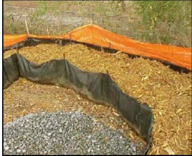
SRB with shredded wood mulch and polymer
