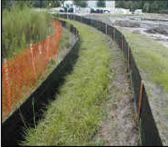
SRB prior to placement of mulch barrier
