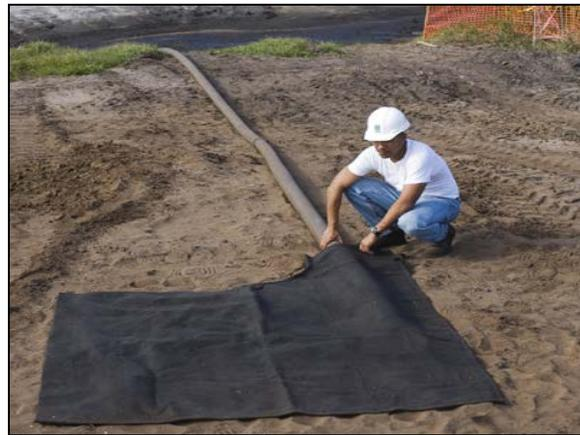
Gravity Bag Filter (Source: <http://www.spillcontainment.com>)
