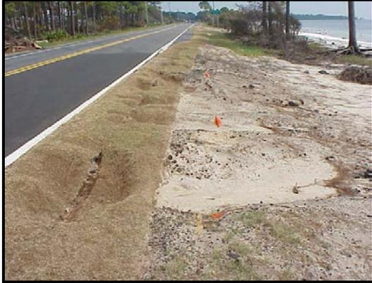
*Evidence on sheet erosion and undercutting of sod, August 2005*
