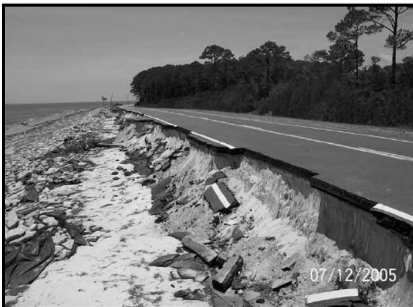
*Front slope and shoulder damage on highway, July 12, 2005*
