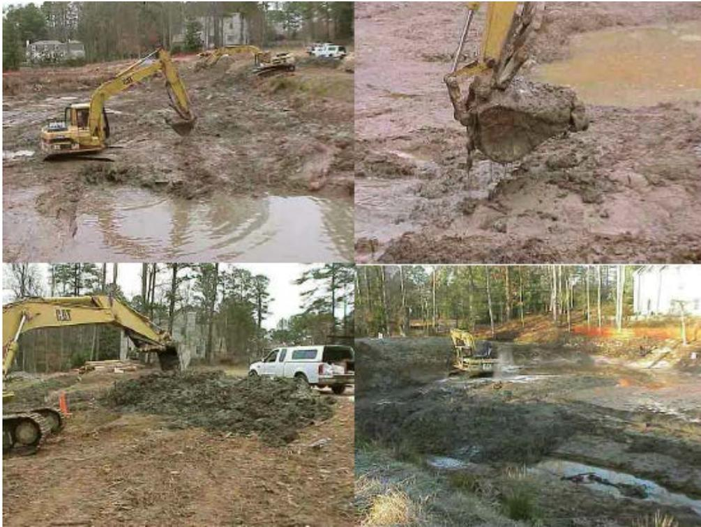
Figure AIII-28: Polymer-enhanced Mud and Sediment Removal.
