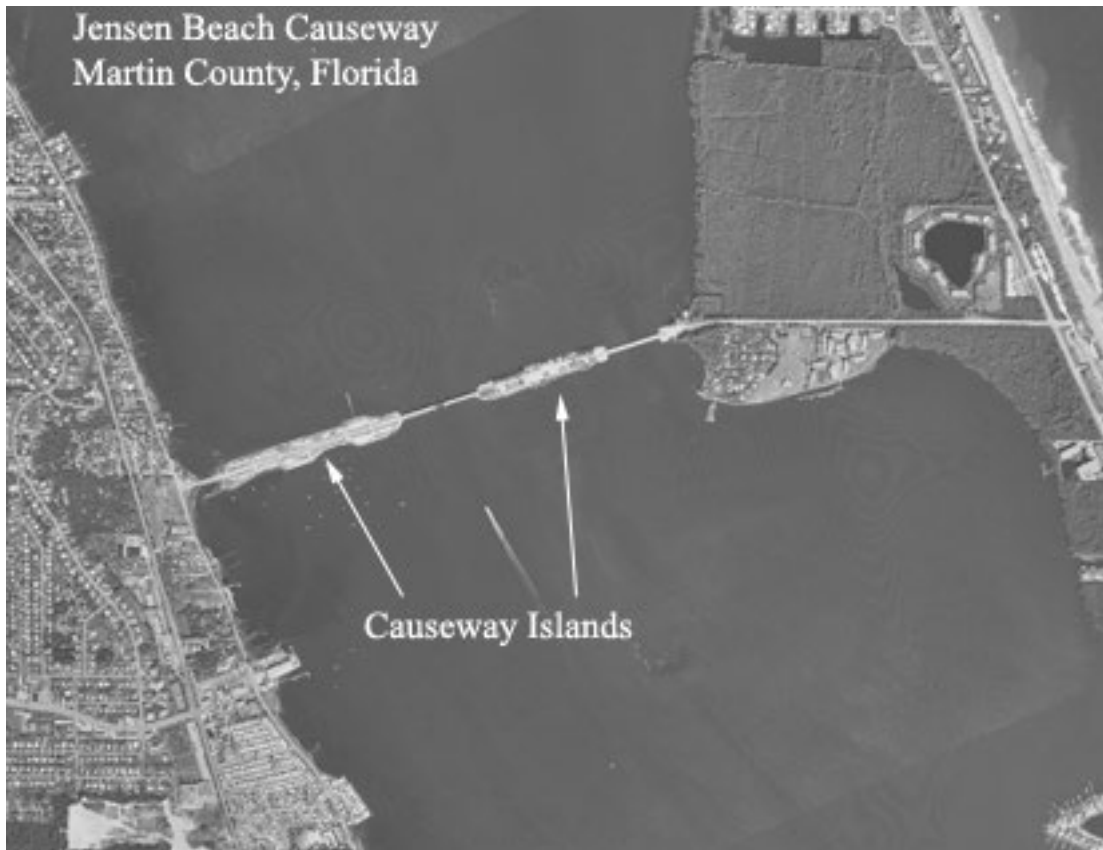
Figure 2-6 An example of manmade causeway islands that create a channel contraction.
