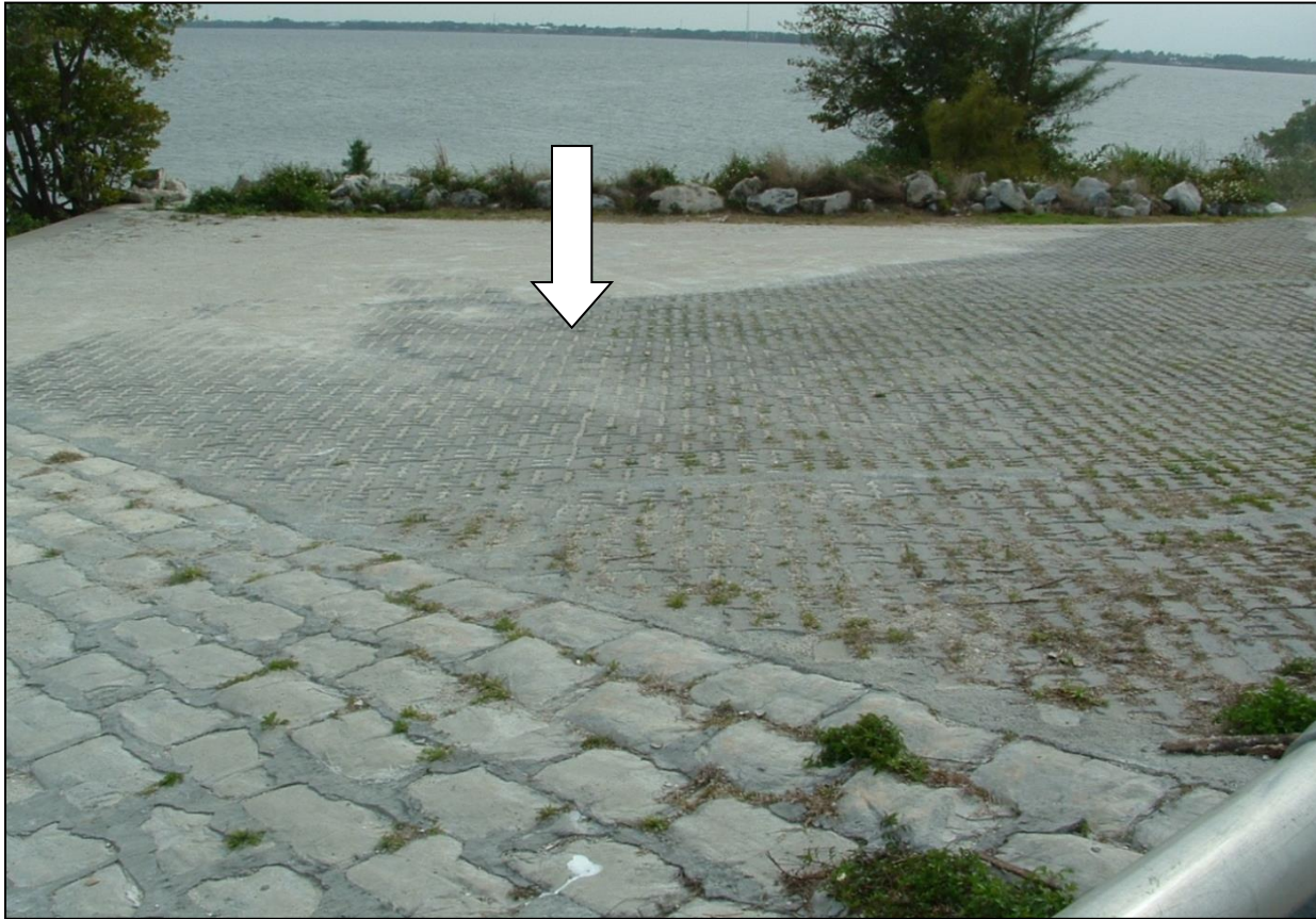
Figure 5.5-14: Example of Articulating Concrete Block Abutment Protection
