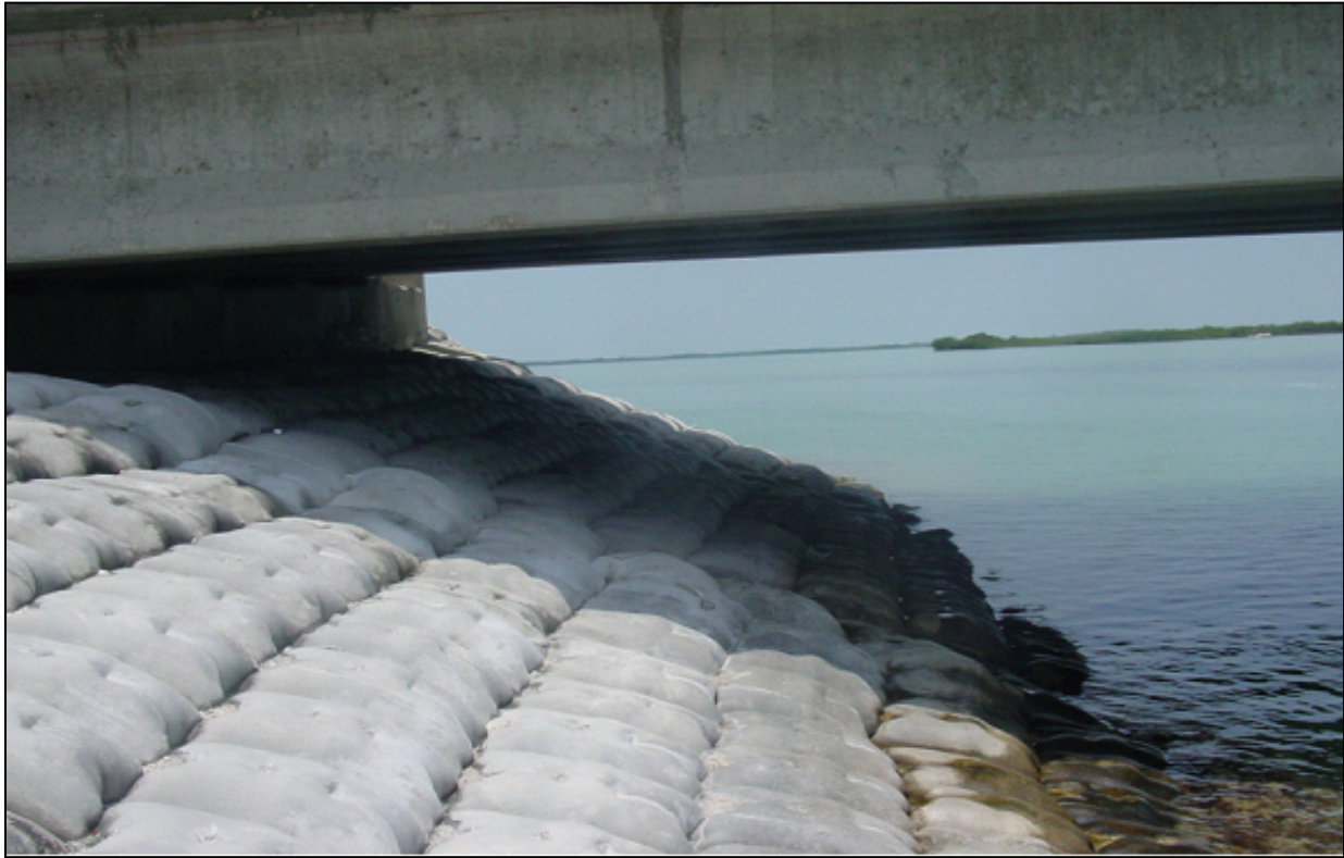
Figure 5.5-15: Example of Grout-Filled Mattress Abutment Protection
