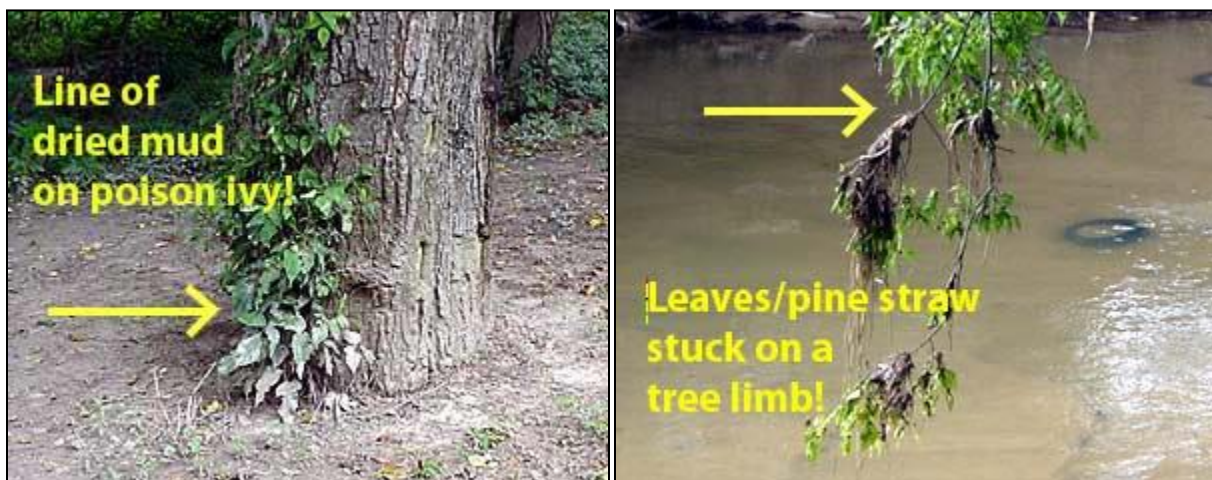
Figure 5.2-21: Examples of High Water Marks after a Flood
