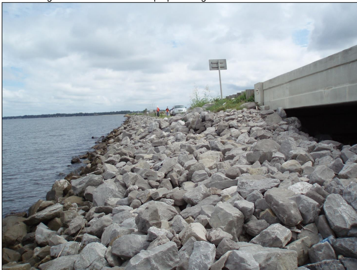
Figure 5.5-13: Example of Rubble Riprap Abutment Protection
