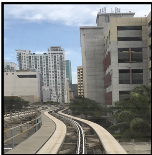
MDT Metromover track
