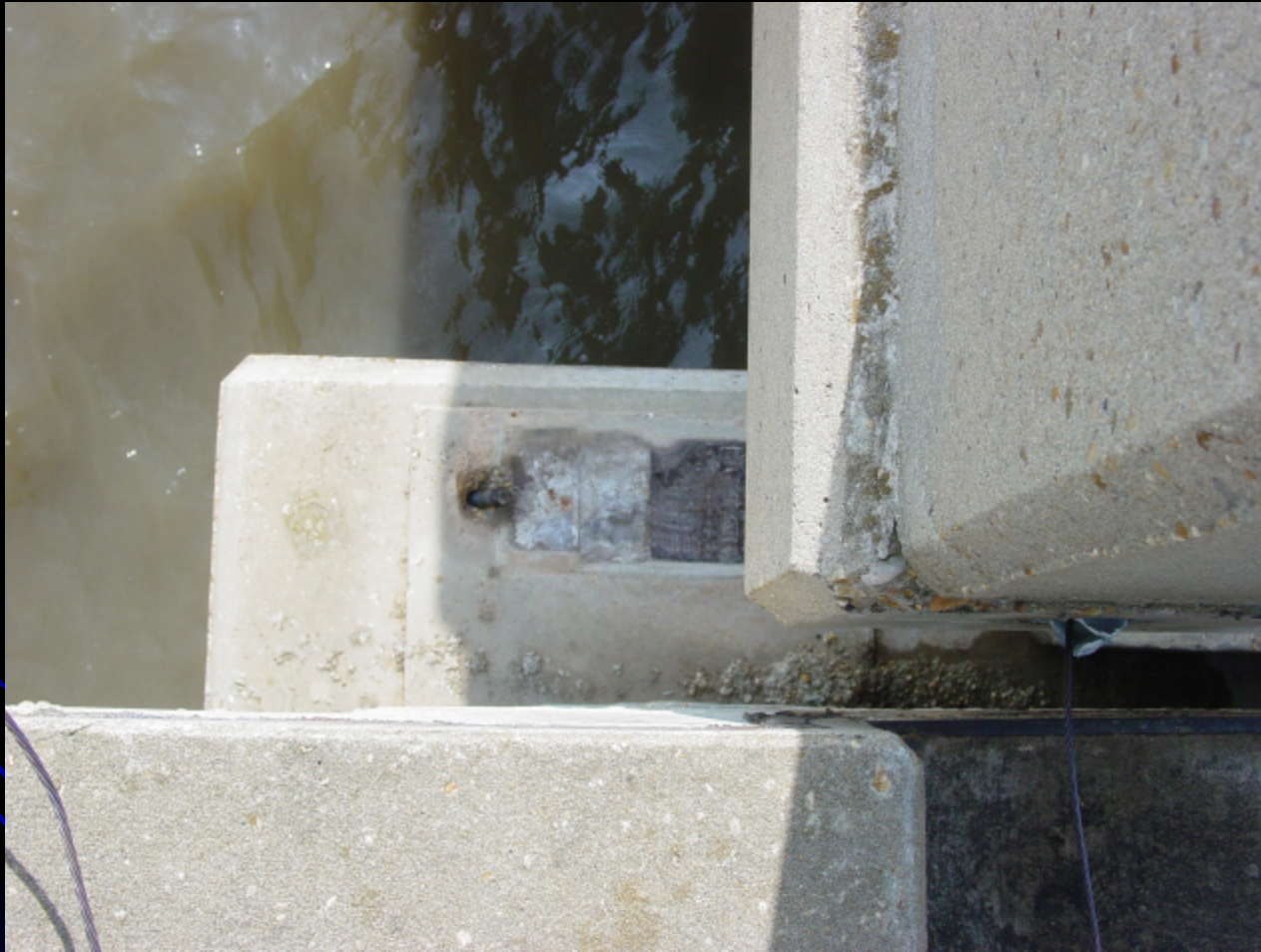
Hold-Down Bolts Sheared
