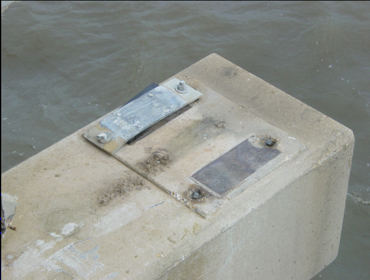
Hold-Down Bolts & Embedded Studs Sheared
