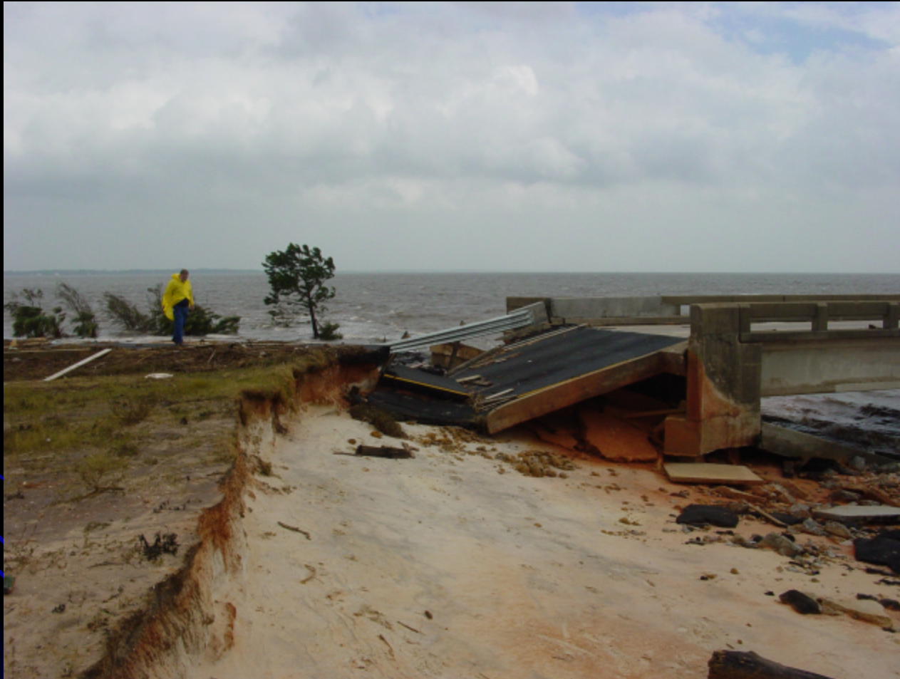
East Abutment of EB Bridge
