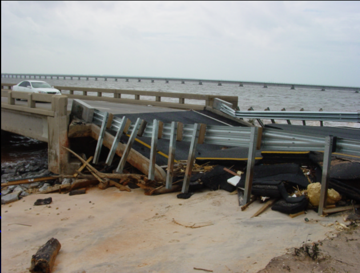
East Abutment of WB Bridge
