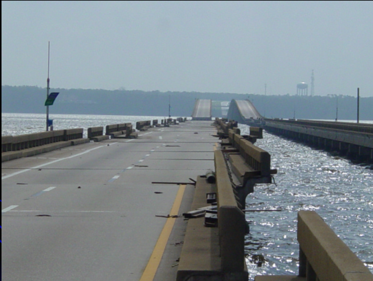
Bridge Looking from East Bank
