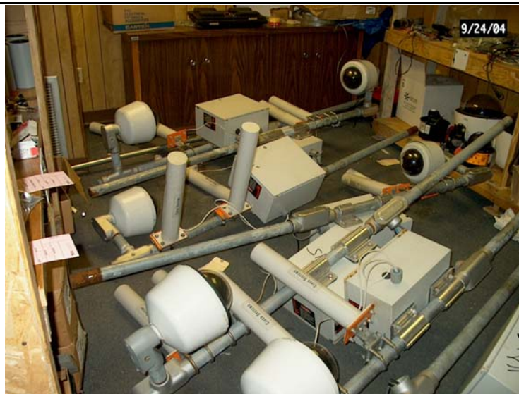
Camera dome assemblies that were removed from SmartZones during Hurricane Jeanne – September 24-26, 2004
