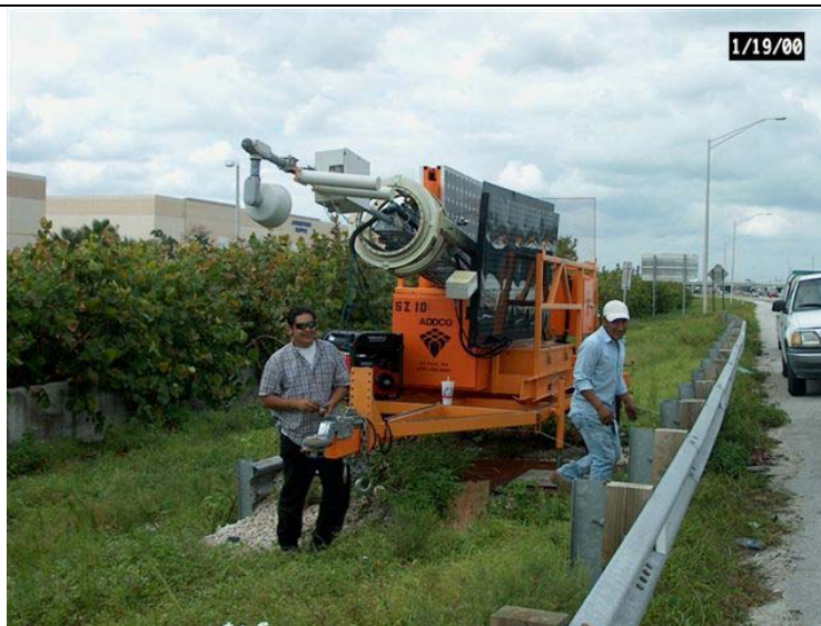
SmartZone #10 retracted prior to dome removal – I-95 southbound south of Palm Beach Lakes Boulevard – West Palm Beach, Florida – September, 24, 2004
