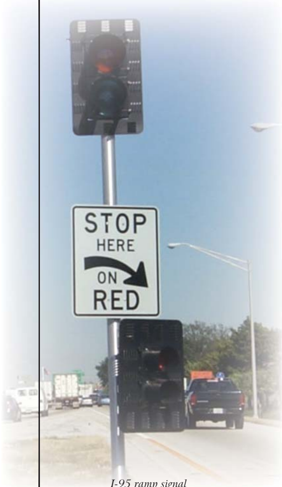
I-95 ramp signal
