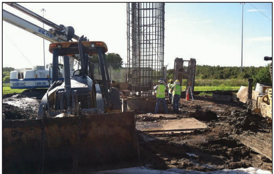
Lowering rebar for steel reinforced concrete drilled pier tower foundations at Canoe Creek Service Plaza.
