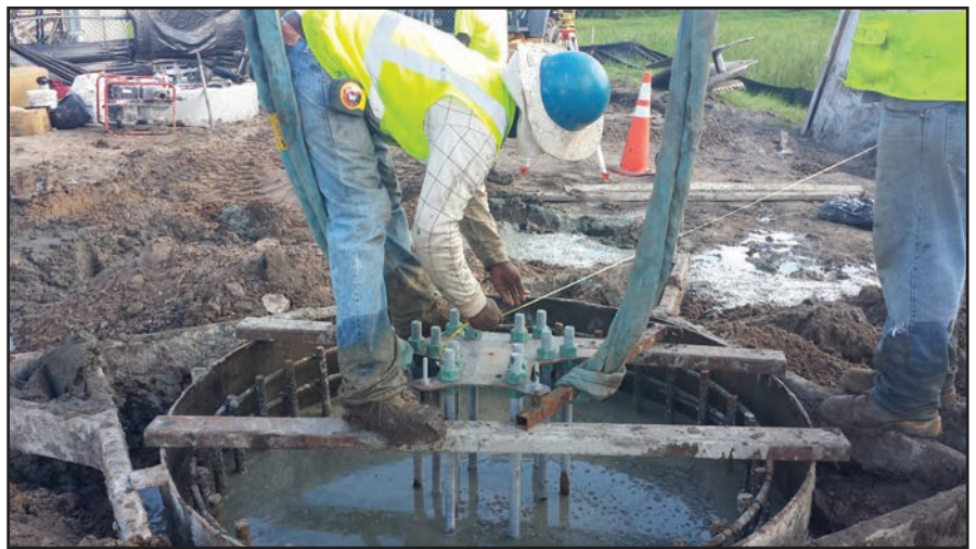
Aligning anchor bolts for drilled pier tower foundation at Canoe Creek Service Plaza.
