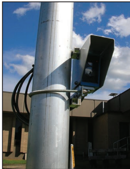
Over-height detector installed at the TERL.
