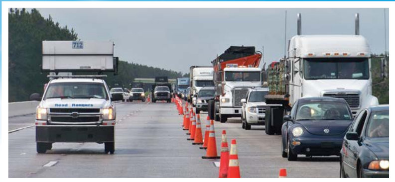
Commercial Vehicle Operations/ Traffic Incident Management
