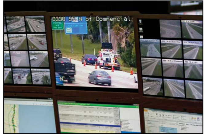
District Four operator console. Photo courtesy of FDOT District Four
