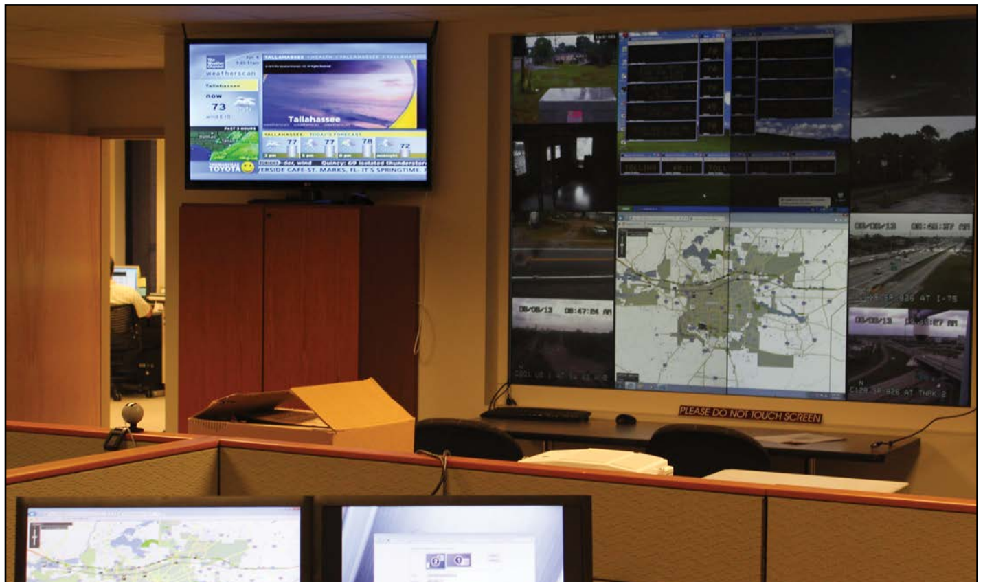
Video wall inside the TERL.
