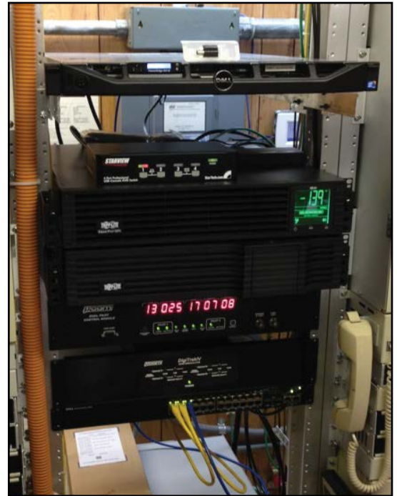
FDOT Satellite Earth Station Receiver Equipment at Lake City.
