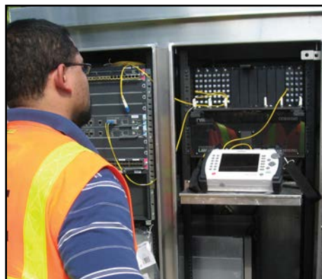
Review systems configuration, technician notes, as-built plans, and wiring schematics in the field. (Photo courtesy of FDOT District Four)
