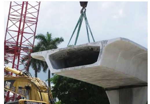
Segments from this decommissioned ramp were used to evaluate non-destructive testing methods.
