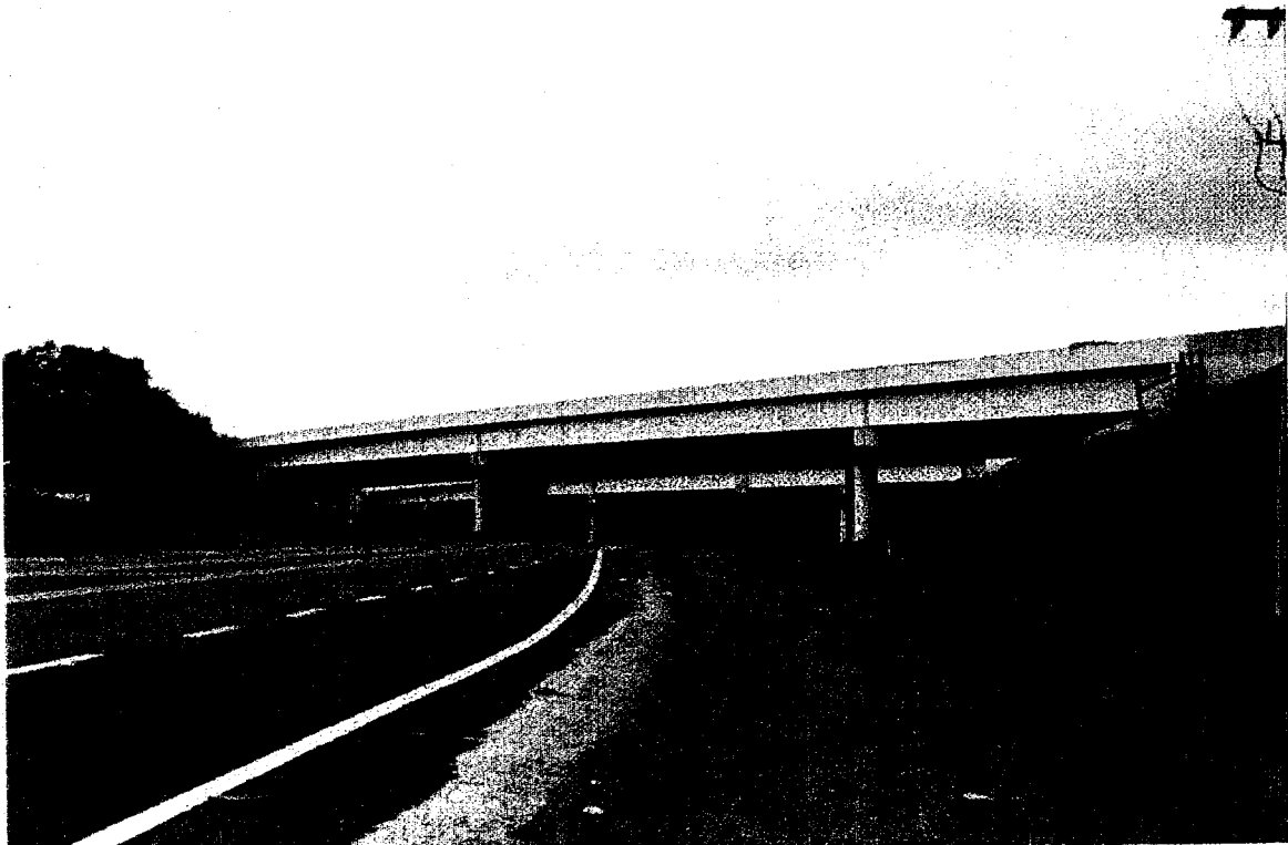
Fig 3.12 Longitudinal view of bridge #100477
