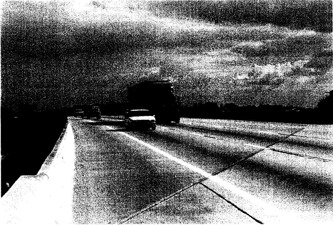
Fig. 3.11 Bridge # 100478 (Northbound I-75 over U.S. 301)
