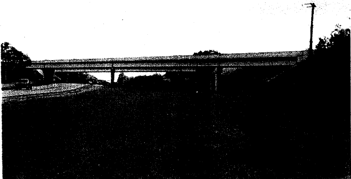
Fig 3.10 Longitudinal view of bridge #100477
