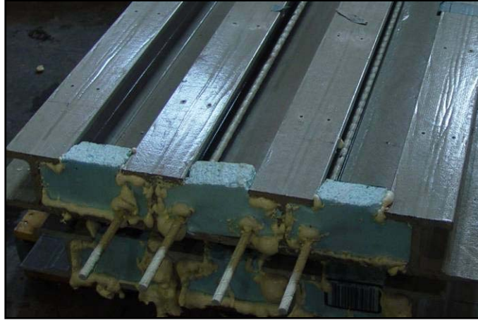
Figure 46 – Bars and foam dams ready for concrete placement
