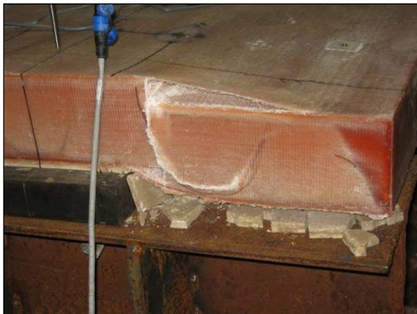
Figure 84 – B_N shear failure over support
