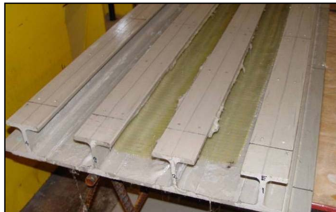
Figure 56 – Partially complete wet layup repair
