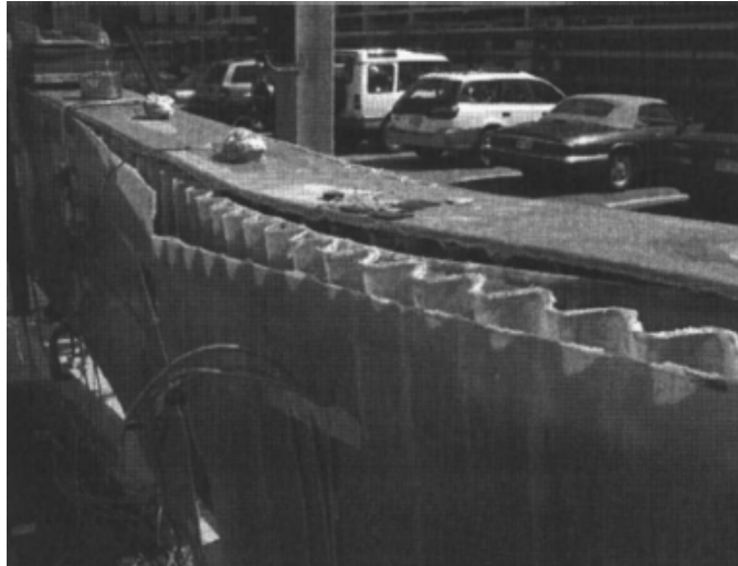
Figure 21 – Picture of the specimen after failure
