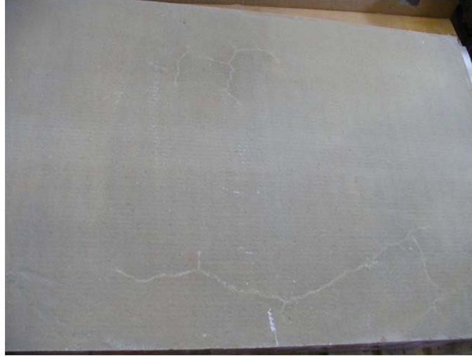
Figure 42 – Specimen B_N wearing surface cracking
