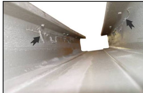
Figure 50 – Specimen A1 web damage before repair
