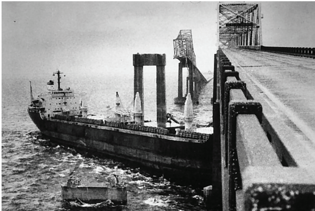
Figure 2.1 Collapse of the Sunshine Skyway Bridge in Tampa, FL (1980) due to ship collision
