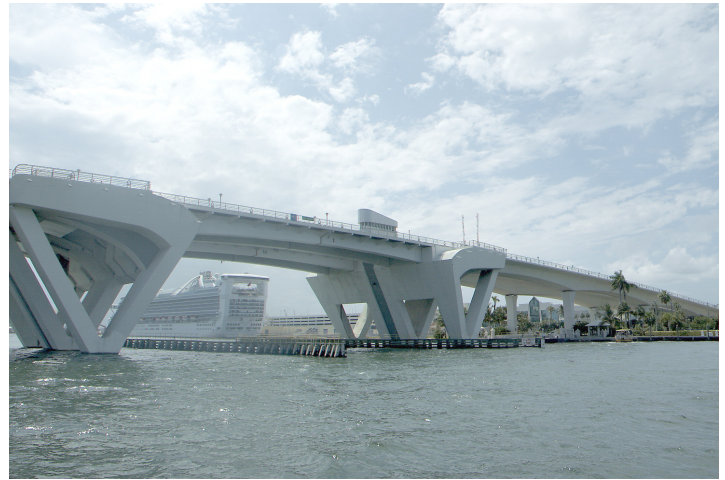
The bascule bridge at SE 17th Street in Fort Lauderdale serves a busy access route for sea-going vessels.
