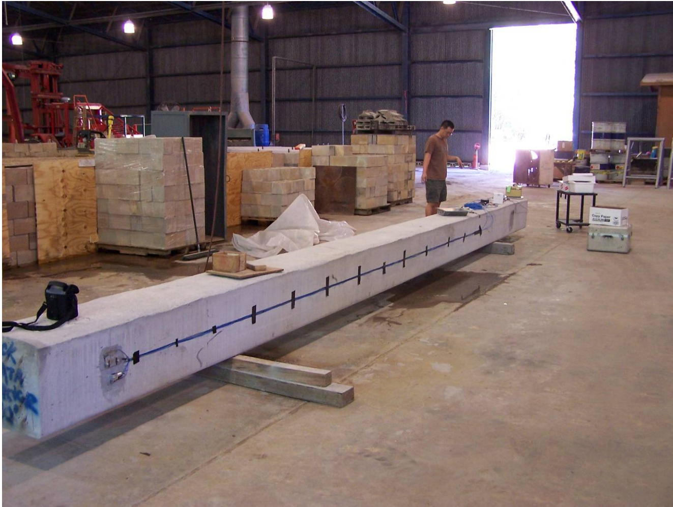
Figure 3-6. Prestressed 18-in \times 18-in \times 30-ft pile with external sensors being attached.
