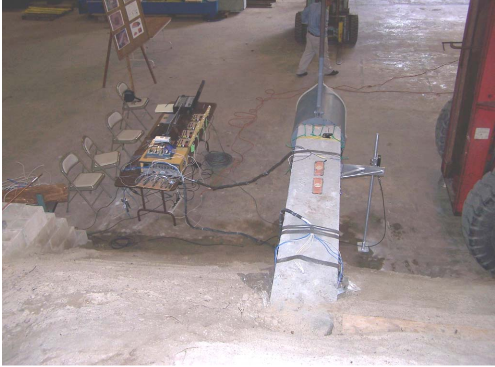
Figure 5-6. Top of 18-in × 18-in × 30-ft exposed 10-ft out of sand embankment.
