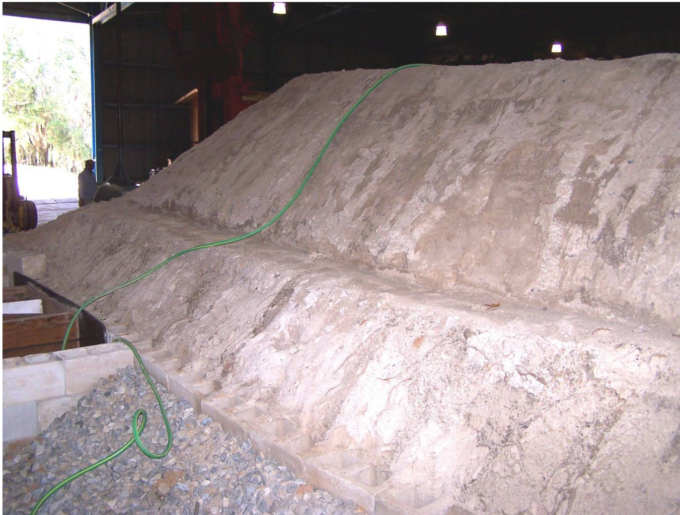
Figure 3-4. Compacted 7-ft high embankment with 18-in \times 18-in \times 30-ft precast pile embedded 20 ft.
