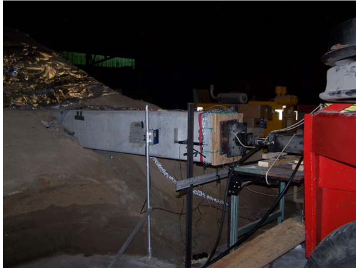
Figure 4-19. Static load test on instrumented pile.
