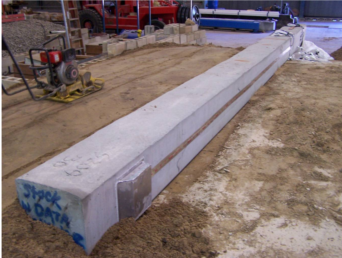
Figure 3-3. Placement of compacted silty-sand adjacent to instrumented pile.
