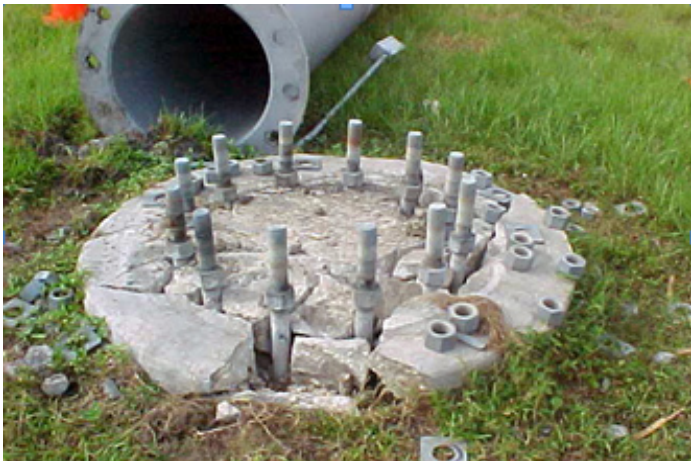
Damaged post base
