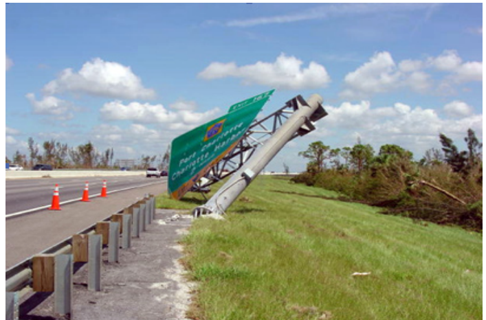
A failed cantilever sign structure
