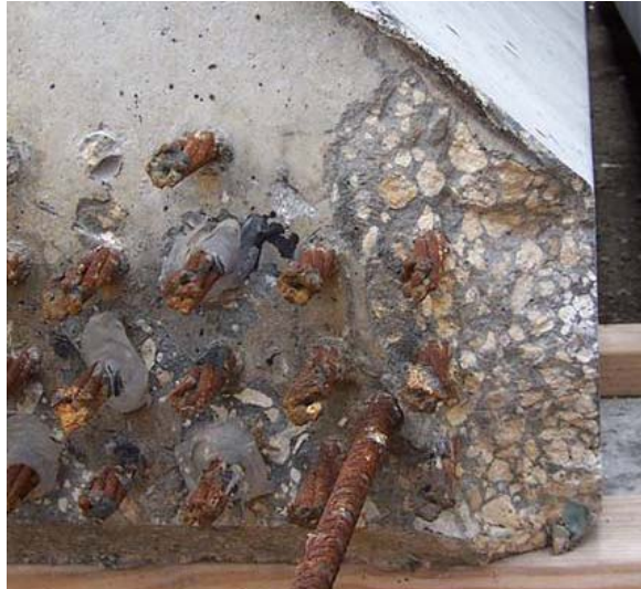
Figure 3-3. Vertical End Crack on Skewed Beam
