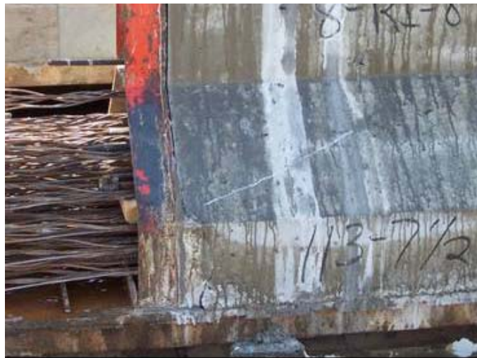
Figure 3-5. Angular Crack
