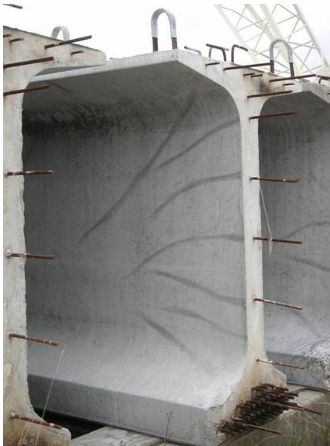
Figure 3-4. Radial Cracking
