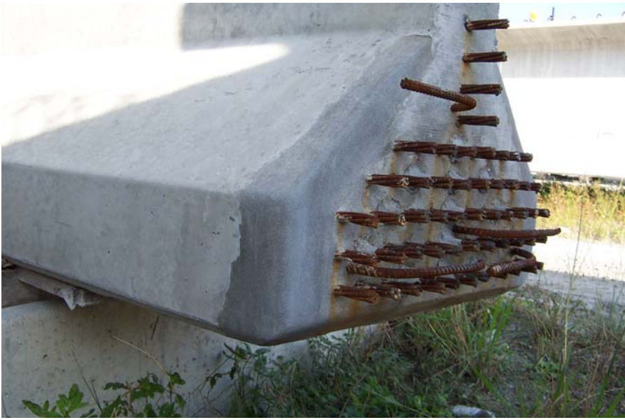
Figure 3-1 Example of Vertical End Crack
