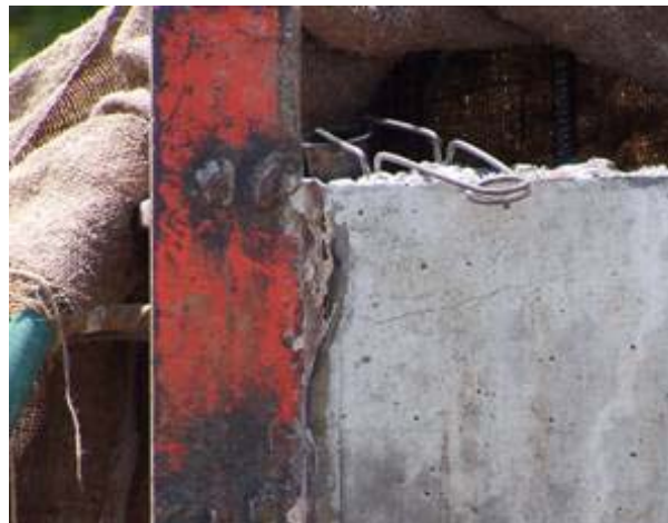
Figure 3-8. Horizontal Top Flange Crack
