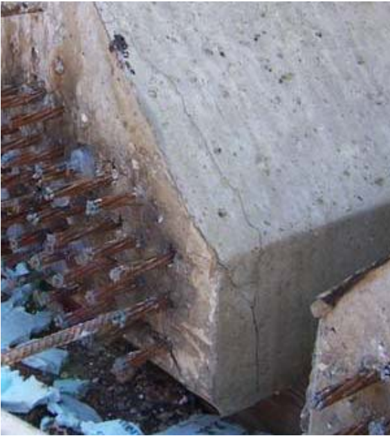
Figure 3-1 Example of Vertical End Crack
