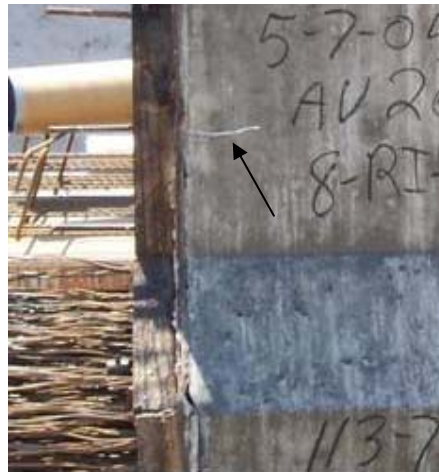
Figure 3-9. Horizontal Web Crack
