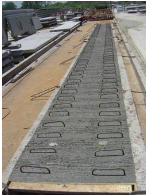
Figure 18. Finished flat slab with hoisting anchors installed
