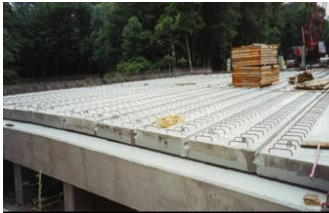
Figure 1. Typical prestressed slab panels
