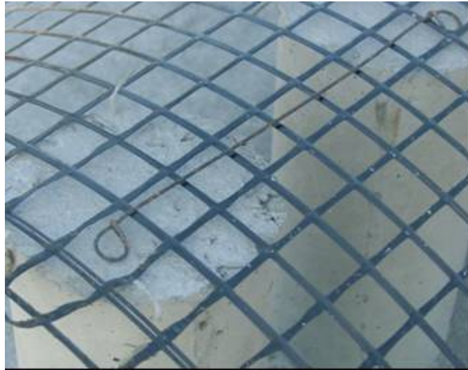
Figure 30. Carbon-fiber grid used in GRD topping
