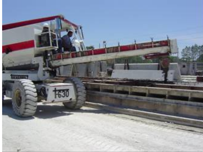
Figure 17. Casting of flat slabs
