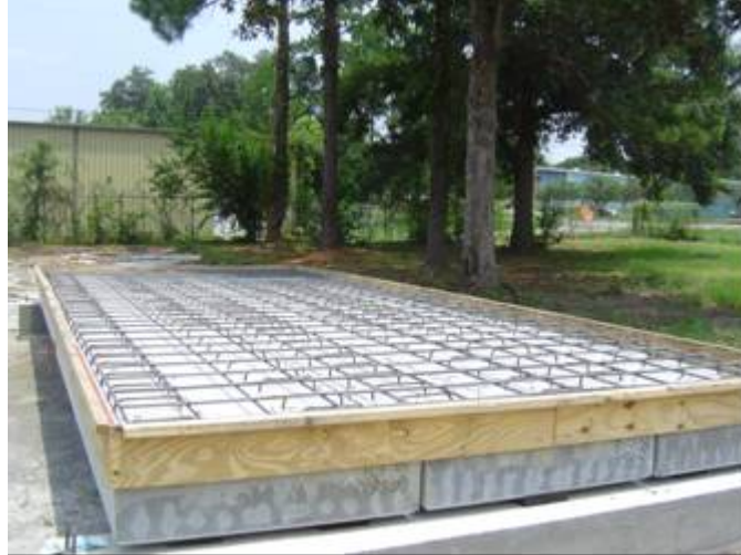
Figure 23. Reinforcement and formwork on precast slabs before topping placement
