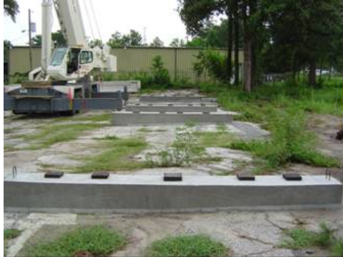
Figure 20. Concrete supports with neoprene bearing pads before placement of precast slabs
