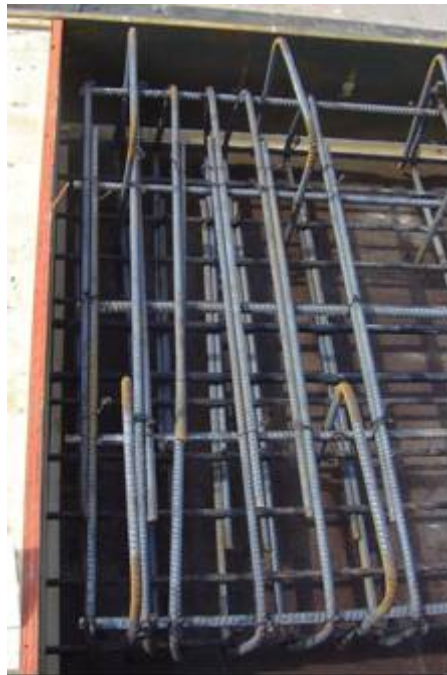
Figure 14. Reinforcement at end of flat slab
