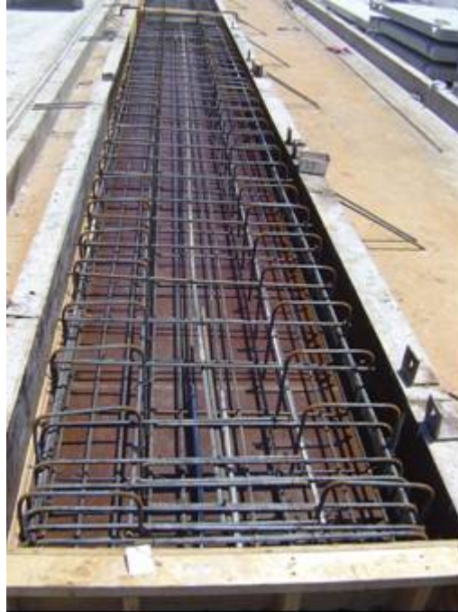
Figure 15. Flat slab reinforcement layout
