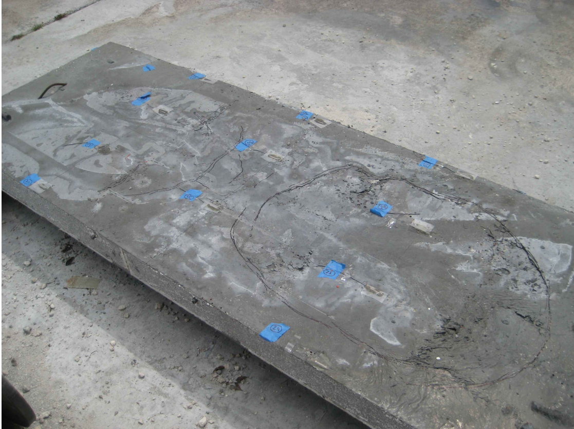
Figure 3.87 Top View of Punching Shear Pattern in Specimen 3T2S
