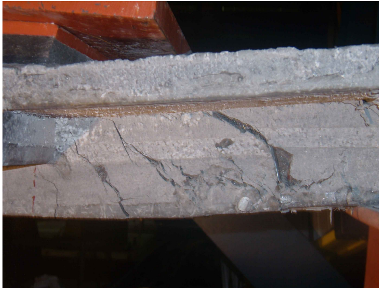
Figure 3.45 Distributed Shear Cracks in Specimen 1T1S with Shear Reinforcement near South Support
