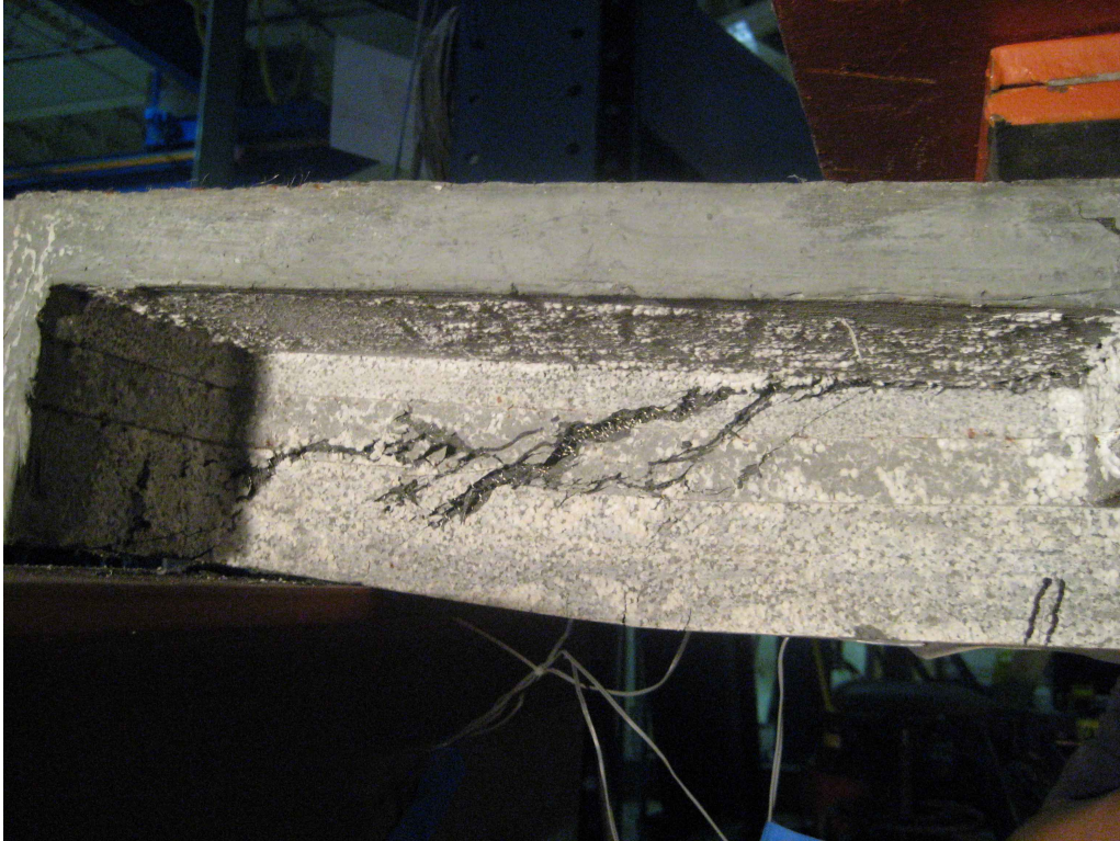
Figure 3.18 Shear-Bond Failure of Specimen 1T1S with End Anchorage
