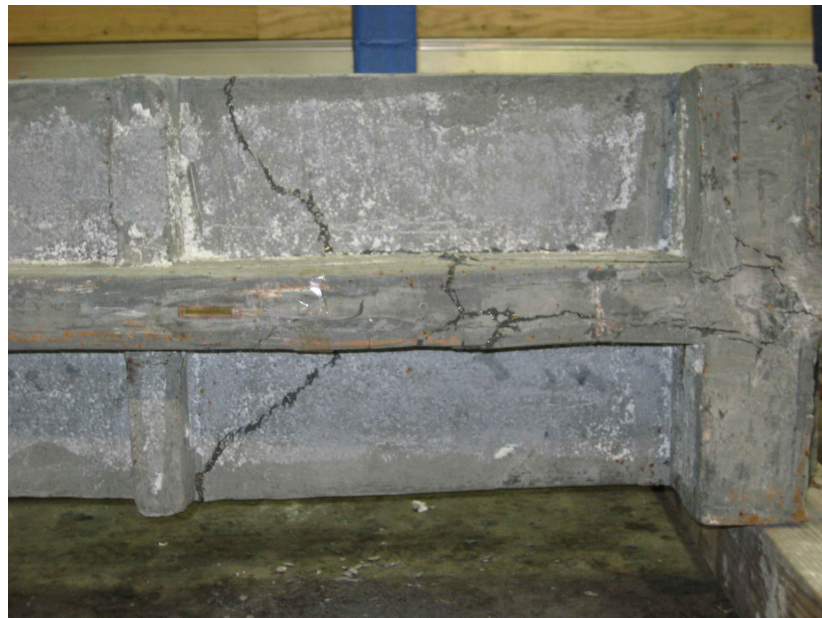
Figure 3.23 Flange Failure in Specimen 1T1S without End Anchorage (Bottom View)
