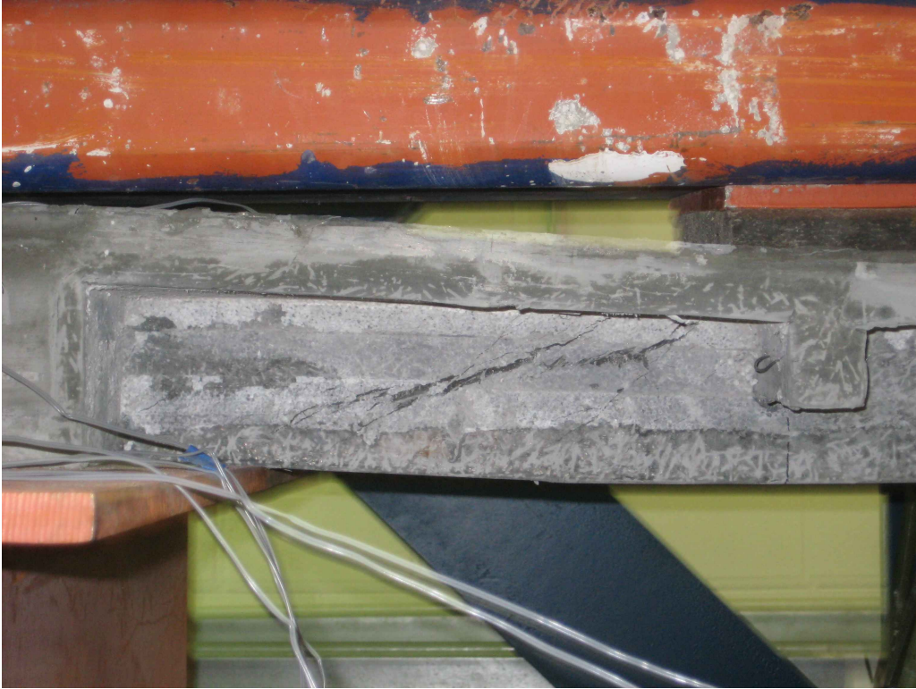
Figure 3.76 Shear Cracks in Specimen 1T2S
