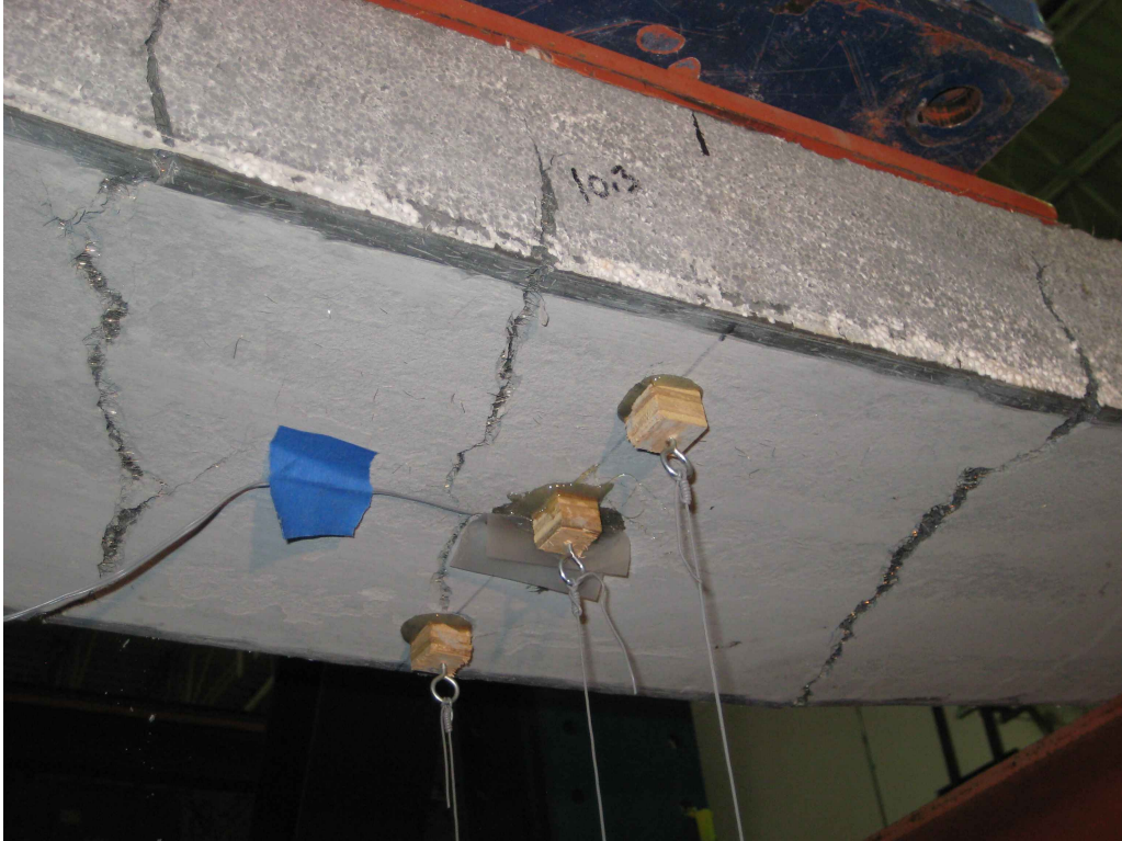
Figure 4.11 Flexural Cracks in the Uniform Section Ductal®-FRP Deck Specimen
