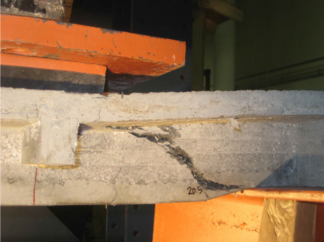
Figure 3.52 Wide Shear Crack in Specimen 1T1S with 1#4 and 2#3 Bent-up Bars
