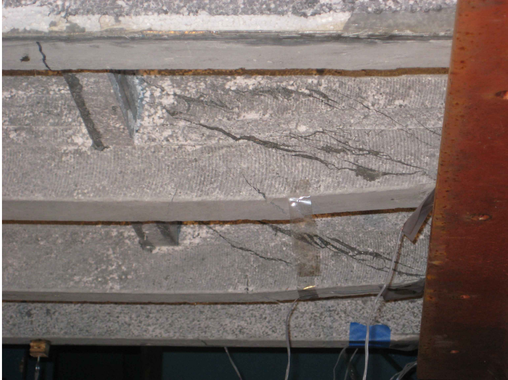
Figure 3.85 Shear Cracks near the Interior Support of Specimen 3T2S
