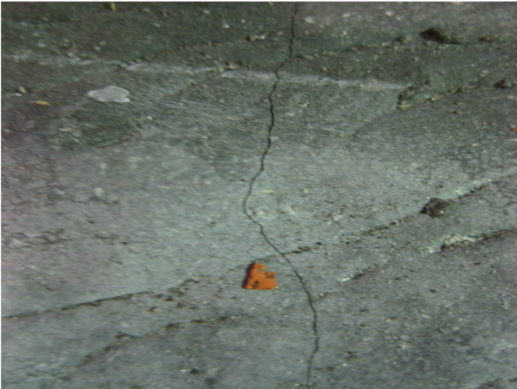
Figure 3.84 Top Flexural Crack at the Interior Support of Specimen 3T2S
