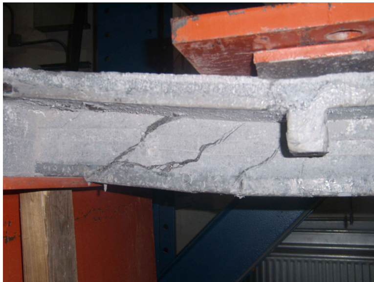
Figure 3.46 Distributed Shear Cracks in Specimen 1T1S with Shear Reinforcement near North Support
