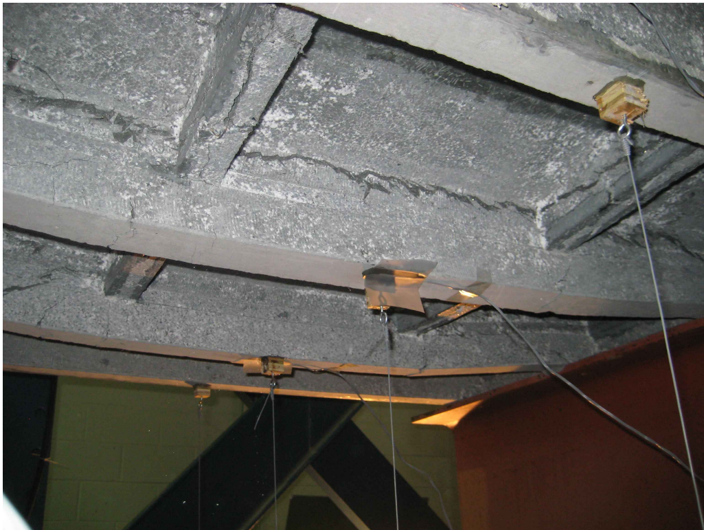
Figure 3.86 Bottom View of Punching Shear Pattern in Specimen 3T2S
