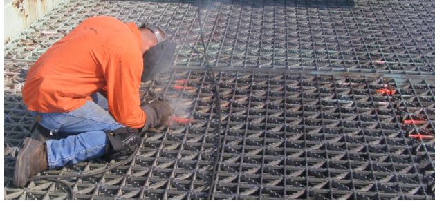
Figure 1.2 Re-Welding of Joints Broken due to Fatigue
