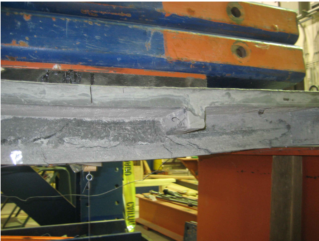
Figure 3.77 Flexural and Shear Cracks in Specimen 1T2S
