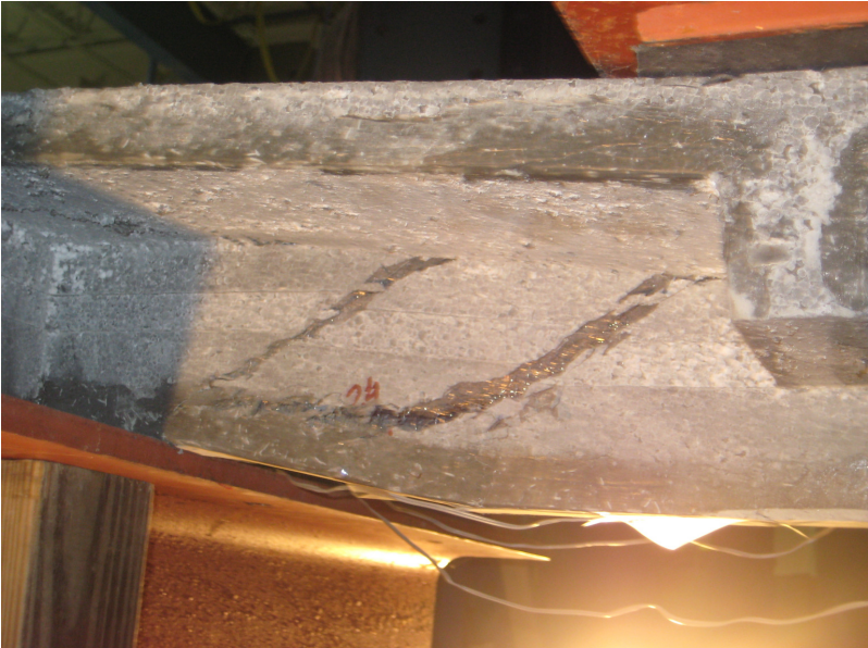
Figure 3.57 Shear Failure of Specimen 1T1S with 2#4 Bars as Flexural Reinforcement
