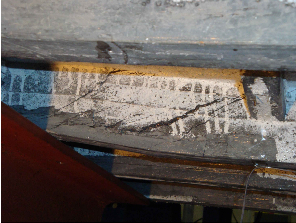
Figure 3.64 Shear Cracks in Specimen 4T1S
