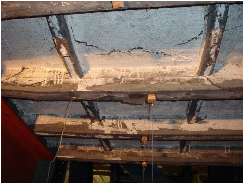
Figure 3.65 Bottom View of Punching Shear Pattern in Specimen 4T1S
