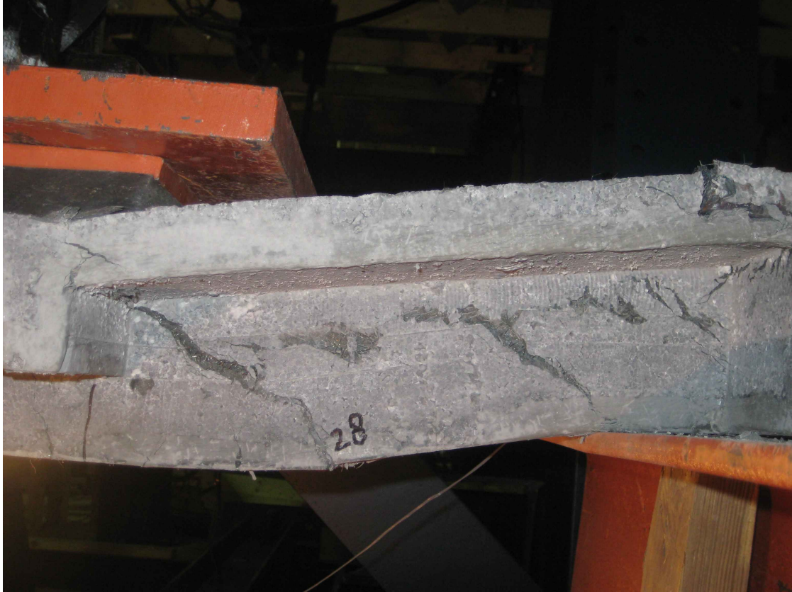
Figure 3.34 Shear Cracks in Specimen 1T1S with 180° Hook near South Support
