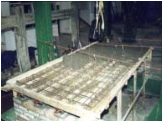
Fig. 4.14 Casting Concrete Slab.
