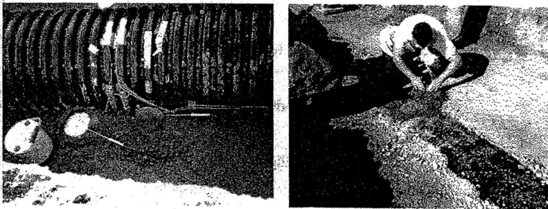
**Fig. 1.2.4 Installation of Pressure Cells**
