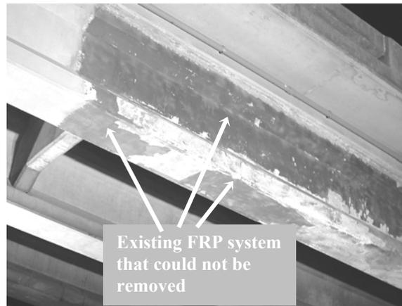
**Figure 19: East girder before new FRP system was applied**
