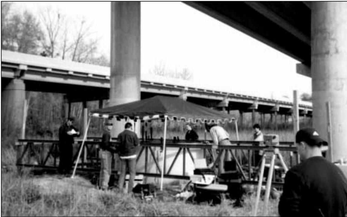
Figure 1.3 Test Setup Overview (Shaft 7)
