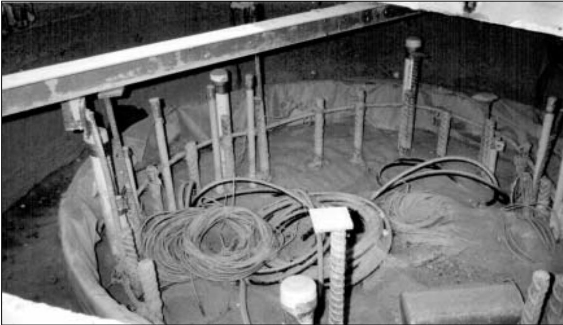
Figure 1.2 Typical Site Conditions Found Inside the Shaft Enclosures
