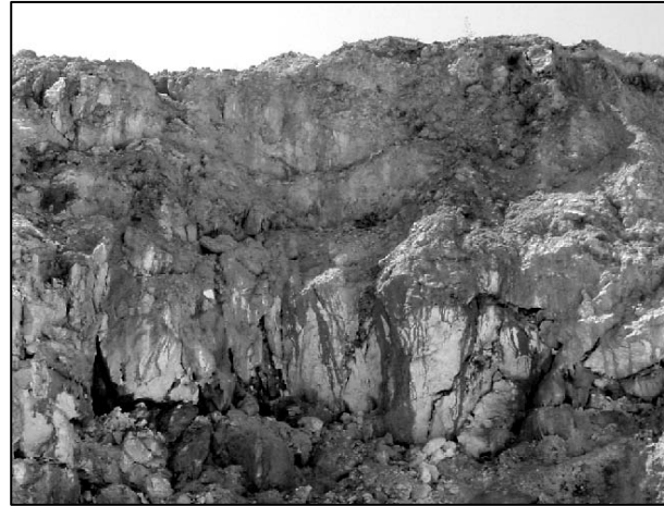
Figure 2.2 Tampa Limestone Exposed in Lecanto, FL Mine
