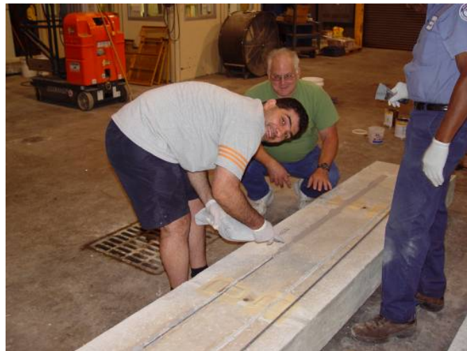
Figure 7 – NSM Bar Installation Using Epoxy.
