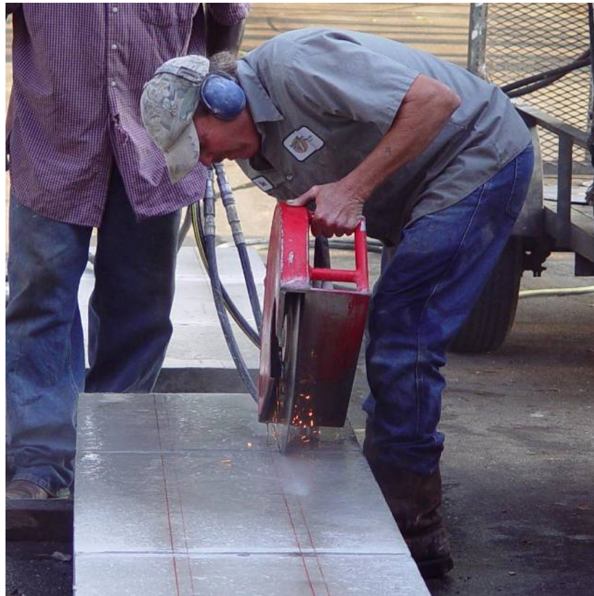
Figure 5 - Groove Cutting.
