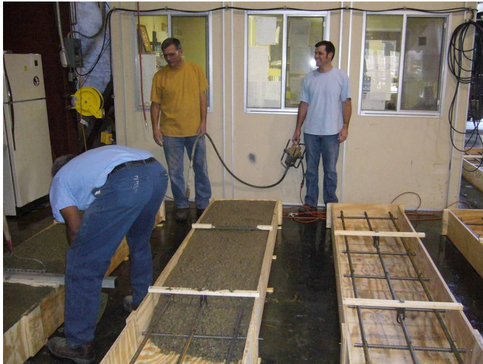
Figure 3 – Casting of Bridge Deck Segments.
