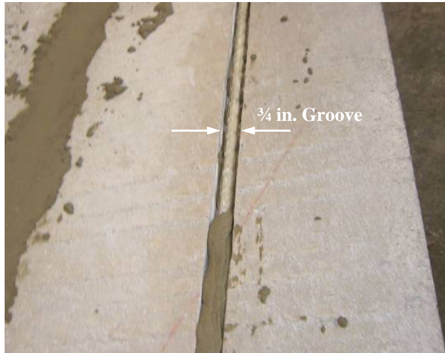
Figure 6 – NSM Bar Installation Using Cement Grout.
