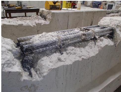
Figure 210—Steel reinforcement exposed
