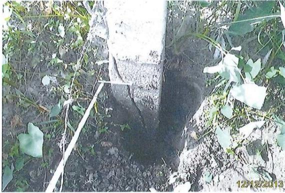
Photo #1 Element 204 - Pile 3-5 fracture in east face
