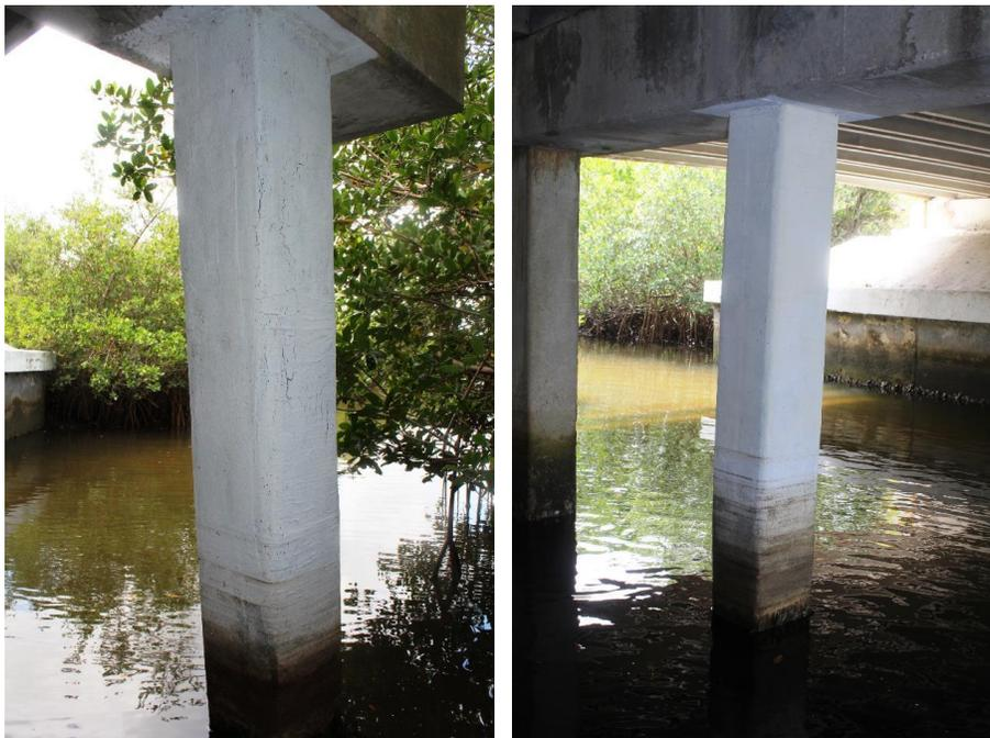
Figure 68—FRP-confined piles on Dickman Road Bridge
