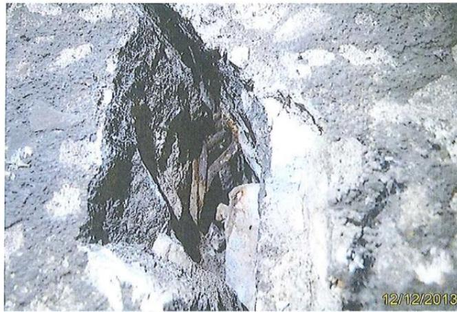
Photo #5 Element 204 - Pile 3-5 exposed and corroded prestress strand (visible through east face)
