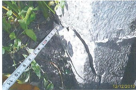
Photo #2 Element 204 - Pile 3-5 fracture in south face
