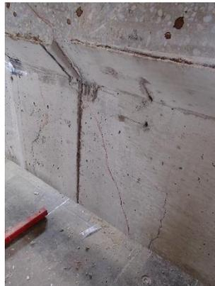
Figure 188—Formwork joint on the east elevation (Girder 5-1)
