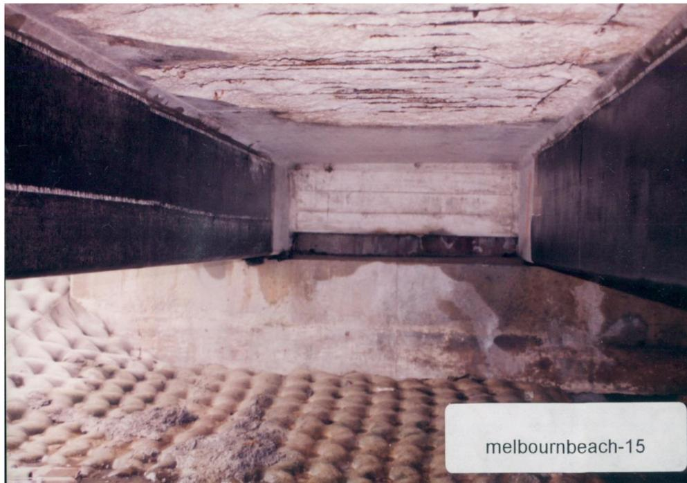
Figure 130—Example of wetting caused by wind and wave action
