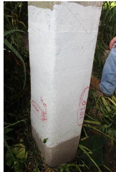
Figure 70—FRP-confined pile on Durant Road Bridge
