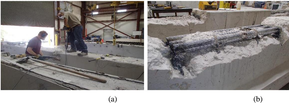
Figure 216—(a) Jackhammering concrete surrounding the reinforcing bars and (b) bridge girder in upside-down position with steel reinforcement exposed
