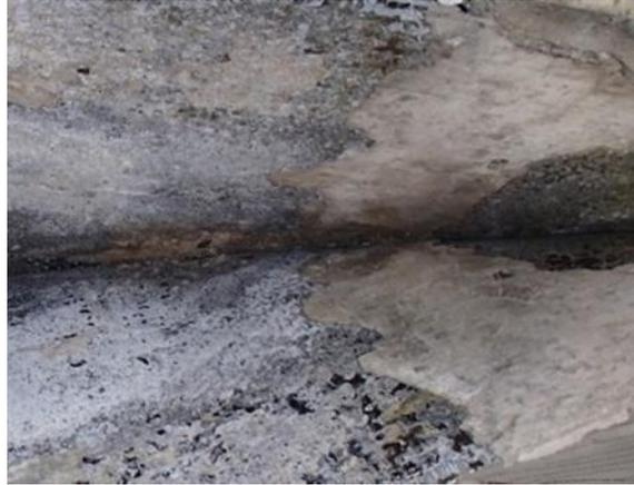
Figure 121—Evidence of skim coat at the bond
