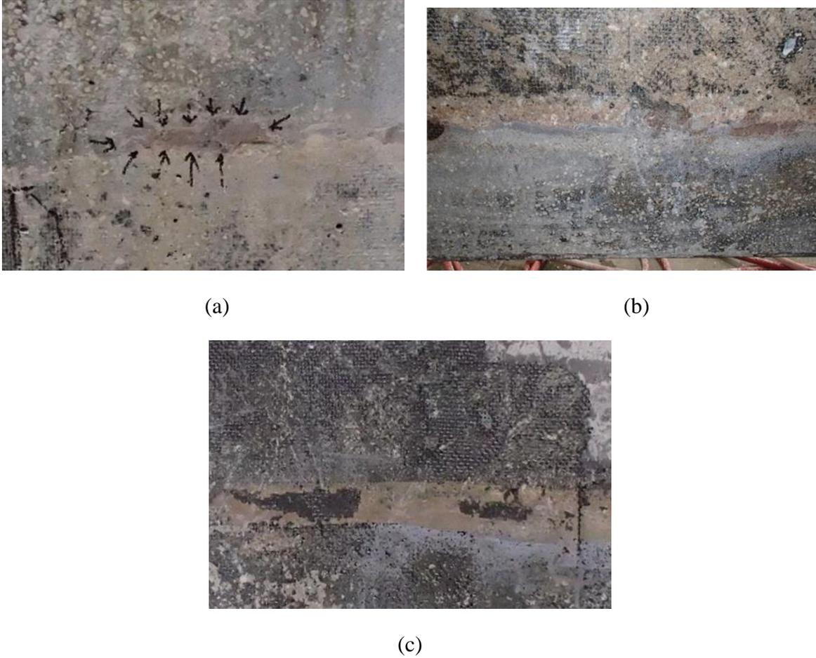
Figure 122—Evidence of primer at the new-old concrete interface
