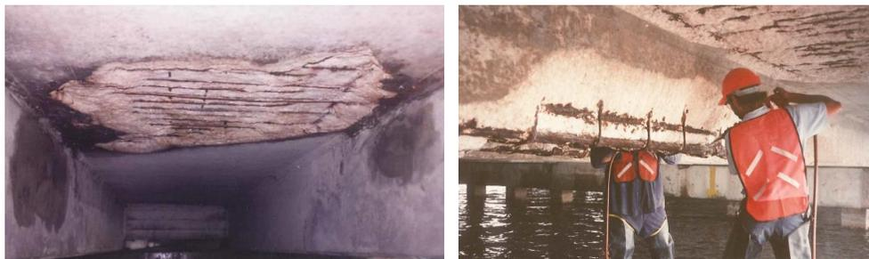
Figure 80—Indian River Bridge – corrosion damage
