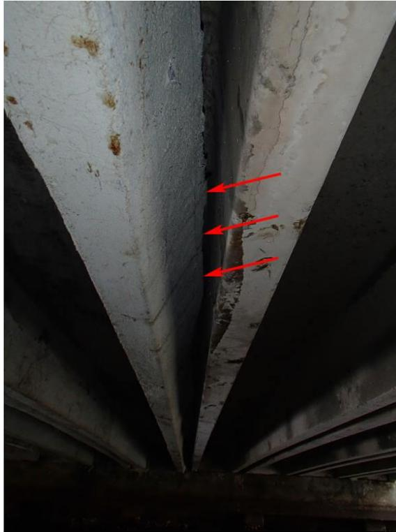
Figure 65—Debonded FRP wrap on a double tee girder
