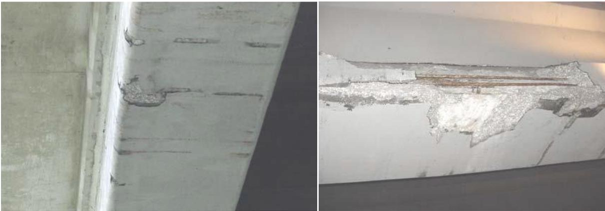
Figure 229—Condition of girder before and after vehicle impact in June of 2003
