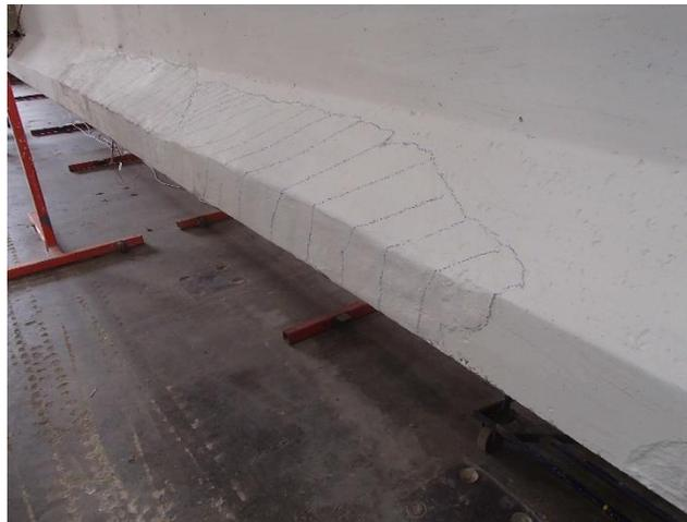
Figure 245—Region of concrete repair indicated in hatched area
