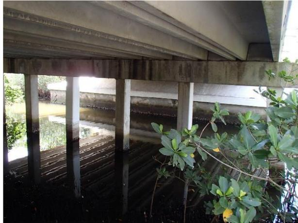
Figure 67—Repaired piles on Dickman Road Bridge
