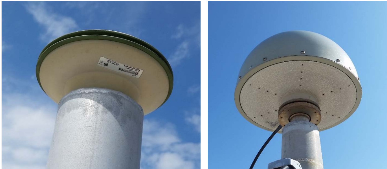
Figure 3-8. GNSS antennae: south end of the main span (left) and center of the main channel span (right).
