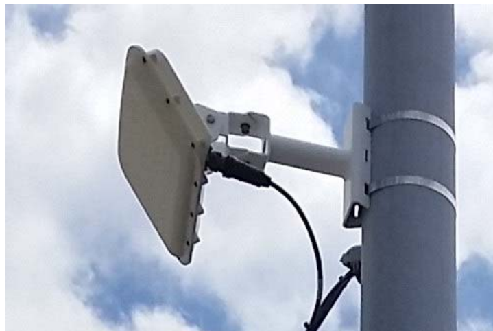
Figure 3-2. The MVDS sensor located at MM 10.6.
