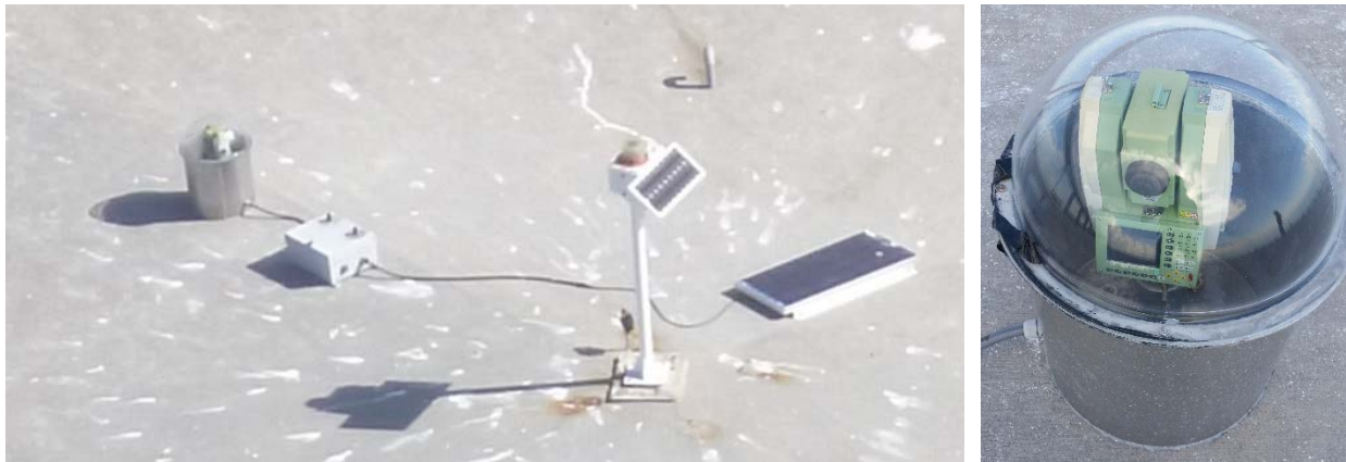
Figure 3-11. Former TM30 AMTS on Dolphin 104 with solar power (left) and close-up (right).
