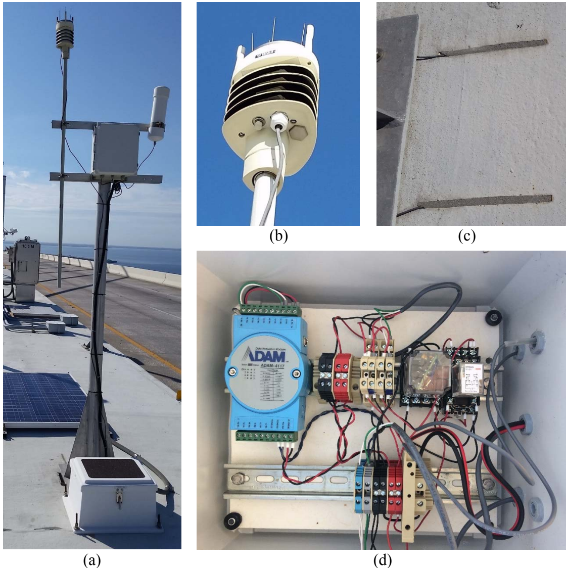
Figure 3-15. (a) Weather station, (b) integrated weather sensor, (c) embedded concrete thermocouples, and (d) interior of the EDS data acquisition and communication box.
