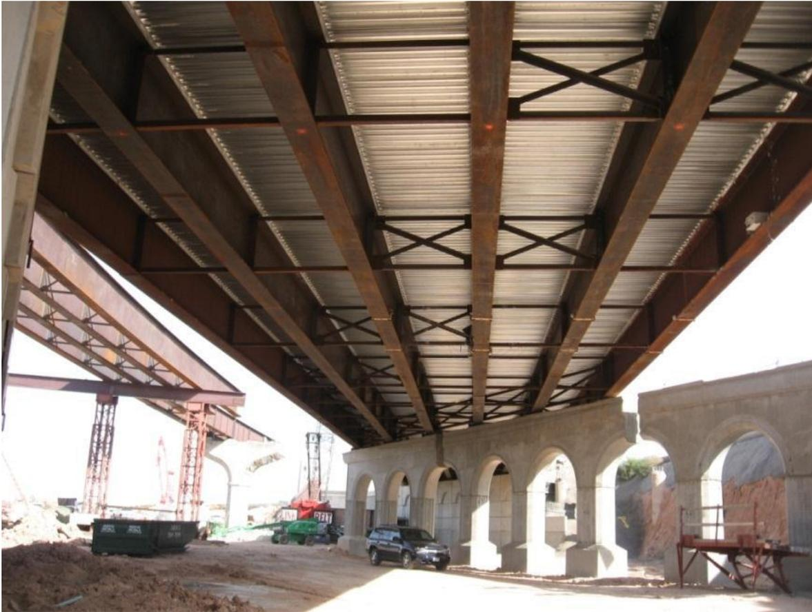
**Figure 5.20: Lean-on bracing system in 19<sup>th</sup> street Bridge**
