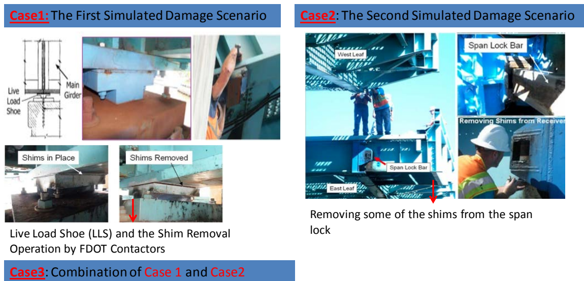
Figure 31 -Implemented damage scenarios on the Sunrise Bridge
