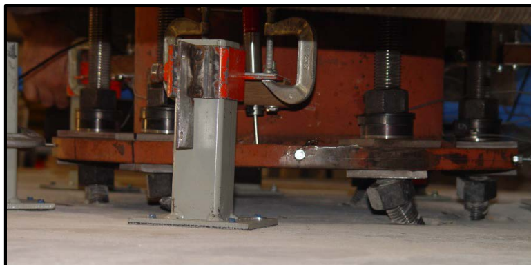
Figure 5-8. FS1 anchor bolts in failed condition
