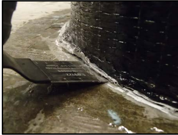
Figure 4-6. Cutting away excess epoxy material after cure
