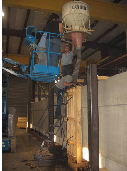
Figure 10.11. Placing concrete into the closure strip formwork
