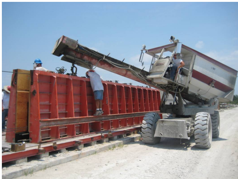
Figure 10.3. Placing concrete in the precast segment formwork
