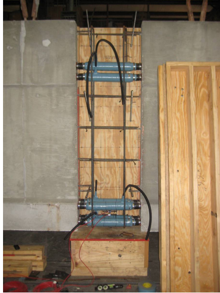
Figure 10.9. Duct couplers in closure strips, sealed with tape prior to concrete placement
