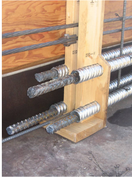
Figure 10.4. Unstressed reinforcing bars placed in ducts to keep ducts straight during placing of concrete
