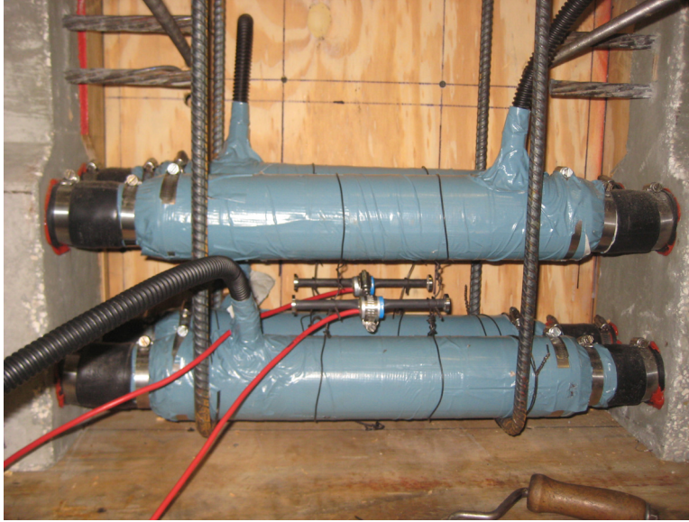
Figure 12.15. Vibrating wire strain gages, cast into closure strips
