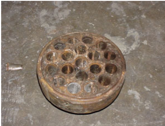
Photo 1 – End View of Anchor Plate
