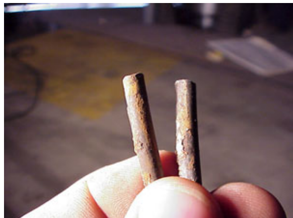
Photo 4 – Close-up Of Pitting Corrosion
