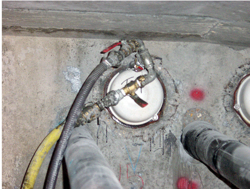
Figure 4.5 – Vacuum injection at anchorages
