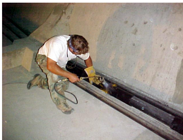
Figure 4.1 – Wrapping External Duct
