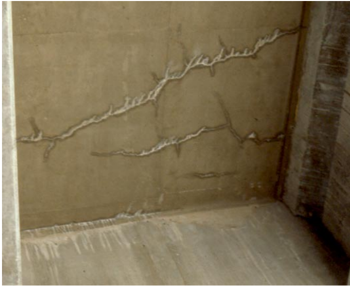
Figure 2.1 – Efflorescence (example - from cracks through a deck slab)
