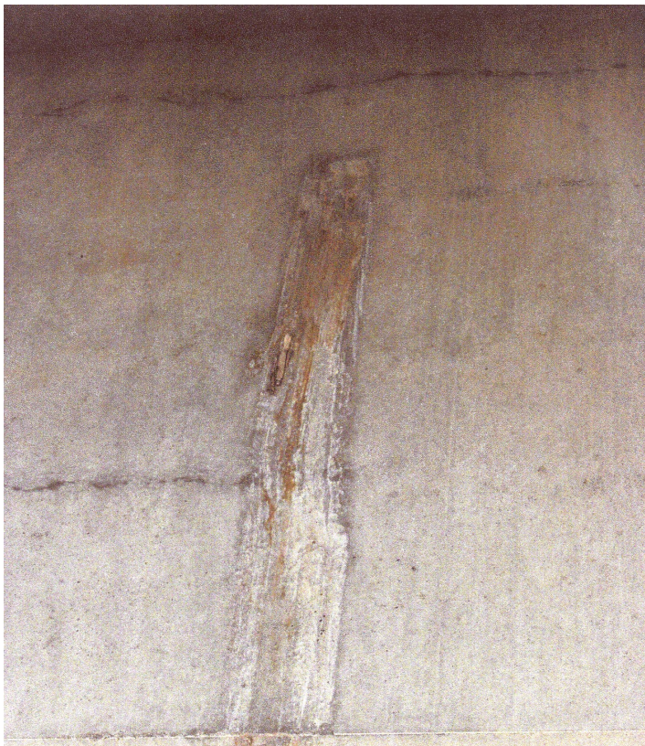
Figure 2.2 – Efflorescence and rust emanating from defect along tendon path in a web
