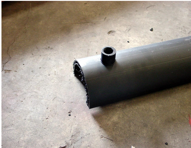
Figure 4.3 – Grout Vent Installed in Half-Pipe Duct
