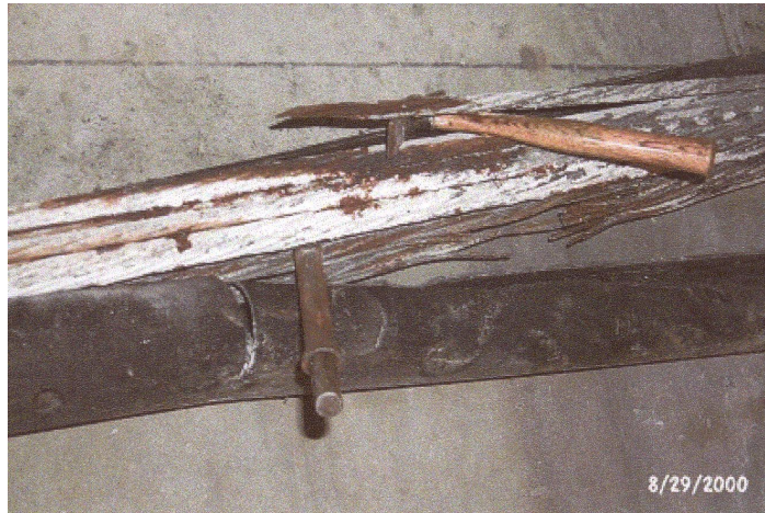
Figure 3.2 – Failure of external tendon due to corrosion (Mid-Bay)
