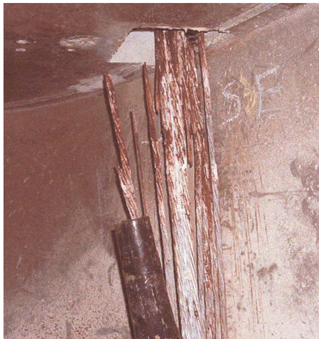
Figure 3.2 – Failure of external tendon due to corrosion (Skyway)
