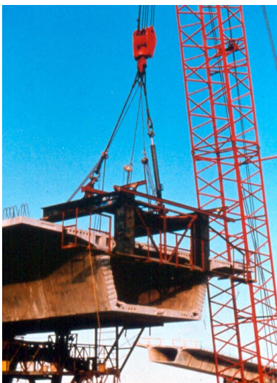
Figure 2.11 – Lifting segments with C-Frame.
