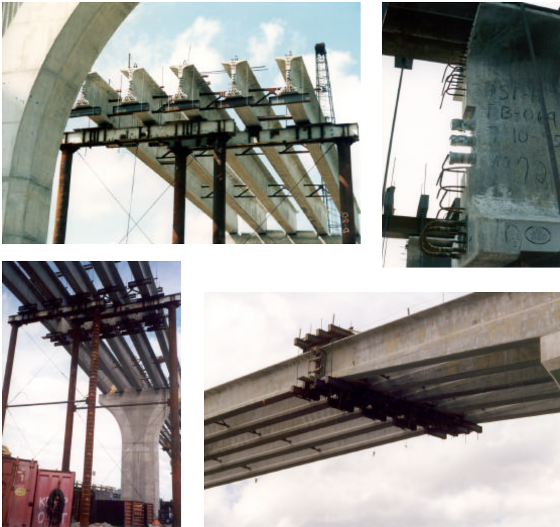
Figure 2.14 – Spliced Girder Main Unit of the Flagler Beach Boulevard Bridge
