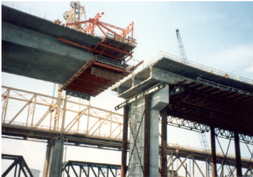
Figure 1.11 – Cast-in-place on Falsework Spans of the Acosta Bridge
