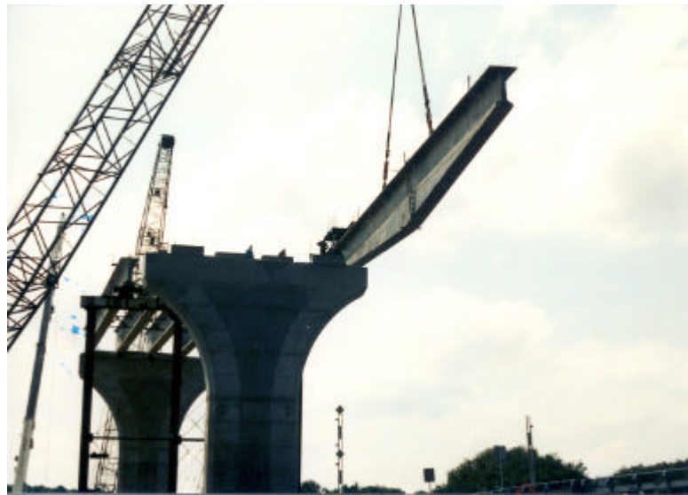
Figure 1.9 – Flagler Beach Bridge, Flagler County
