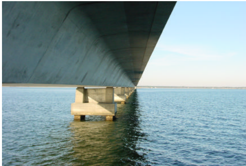
Figure 1.16 – The Mid-Bay Bridge
