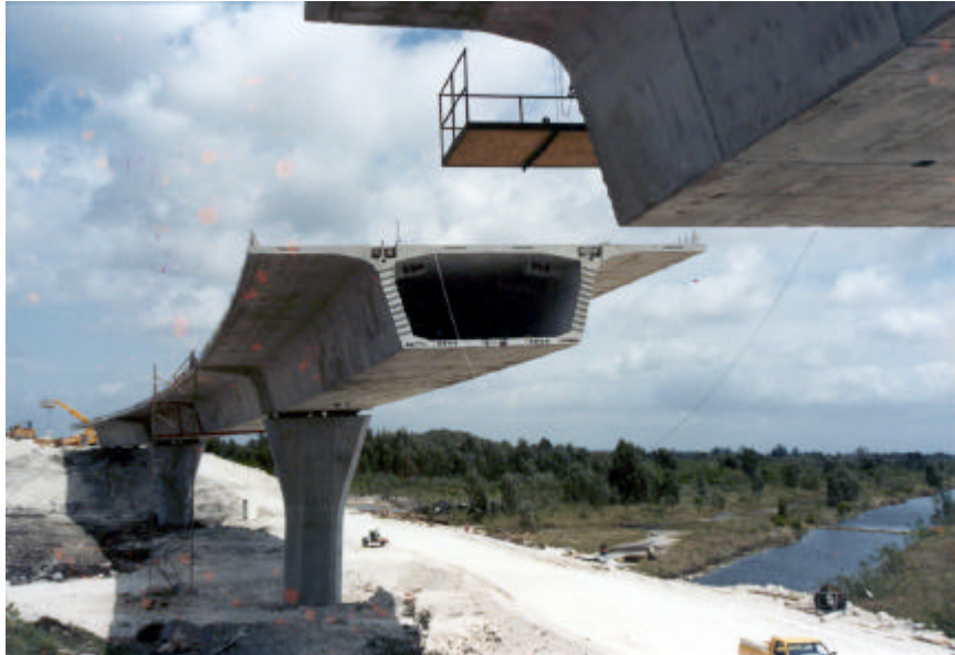
Figure 1.5 – Ramp I Bridge
