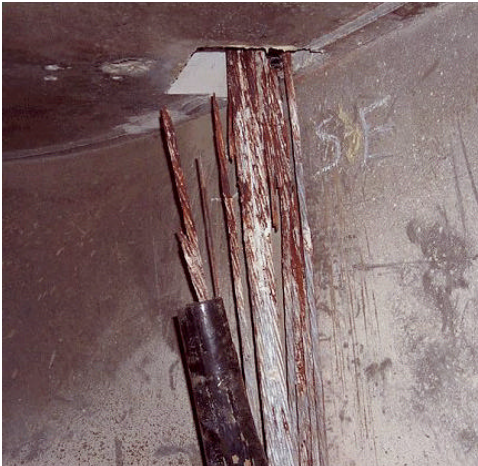
Figure 1.19 – Tendon Corrosion in the Sunshine Skyway Bridge Piers
