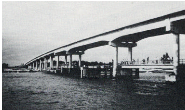
Figure 1.1 - Sebastian Inlet Bridge
