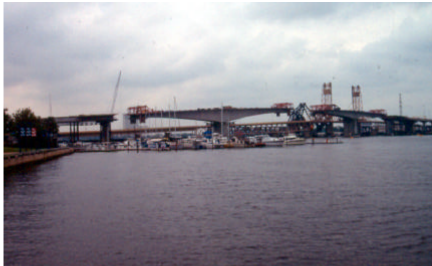
Figure 1.10 – Acosta Bridge in Jacksonville, Florida
