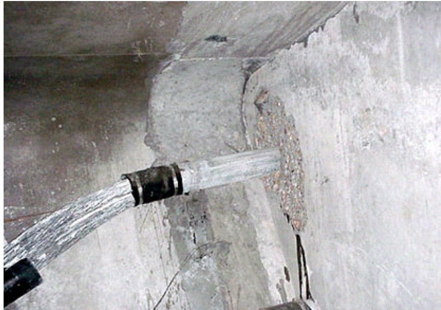
Figure 1.18 – Failure of Tendon 57-1 on the Mid-Bay Bridge (At Expansion Joint Diaphragm)
