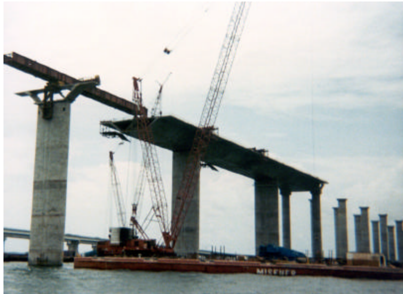
Figure 1.6 – Balanced Cantilever Side Spans of the Sunshine Skyway Bridge
