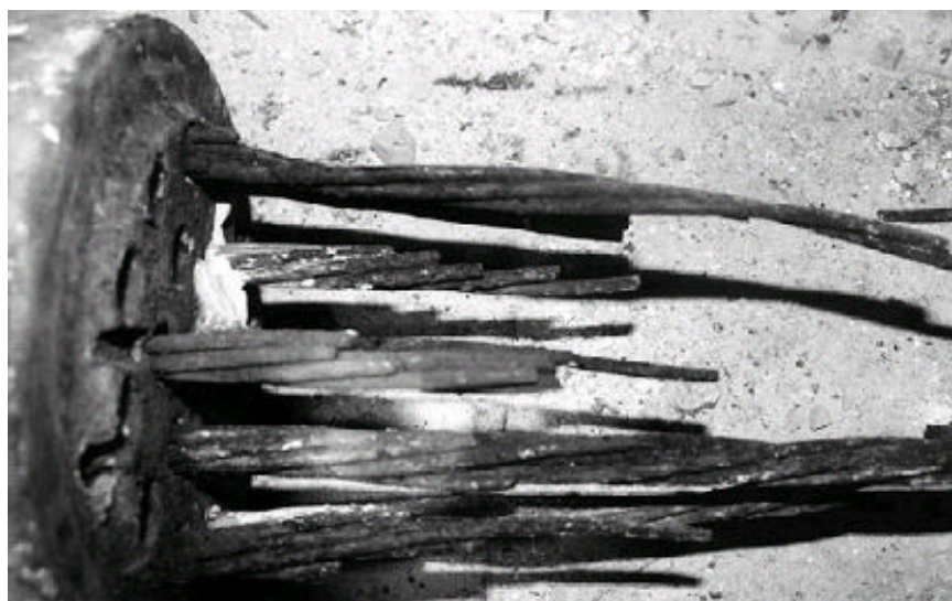
Figure 1.14 – Advanced Corrosion of Strands within Niles Channel Anchorage
