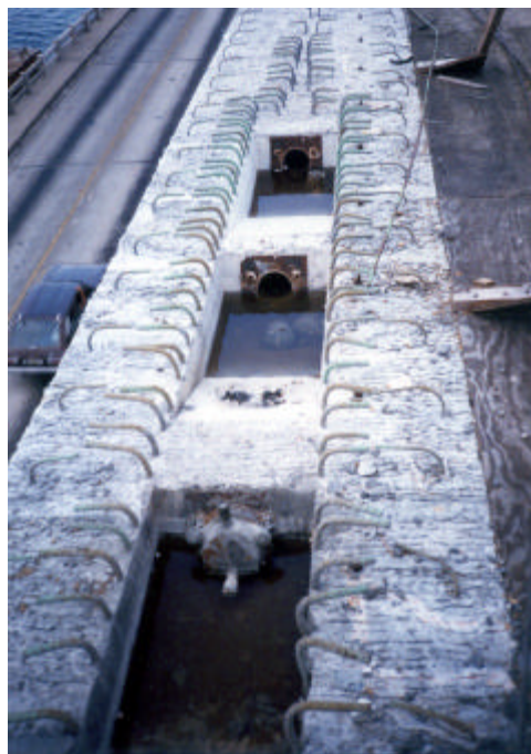
Anchors at Beam End
