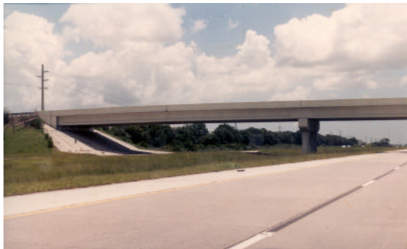
Figure 1.3 – Chipola Nursery Road Bridge over I-10
