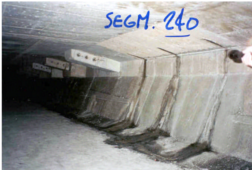
Figure 1.12 – Epoxy Joint Leaking in the I-595/I-75 Interchange
