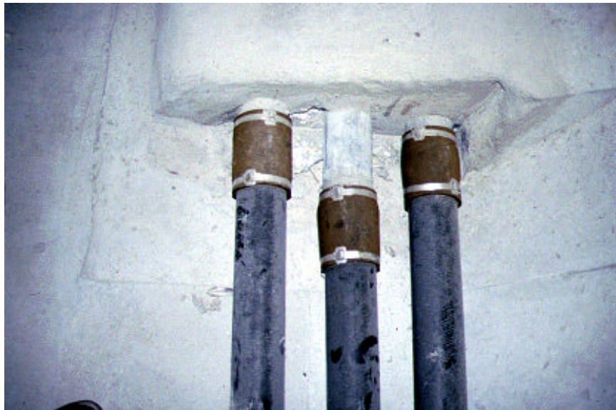
Figure 1.13 – Plan View of Slipped Tendon at Deviation Saddle
