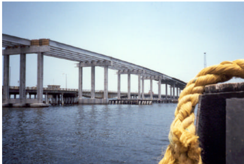
Figure 1.8 – Eau Gallie Bridge
