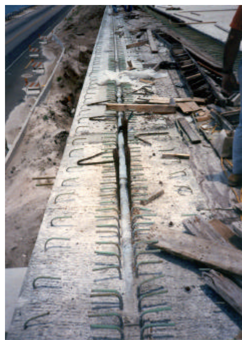
Rising Ducts at Piers
