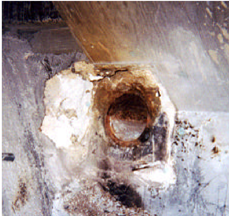
Figure 1.15 – Anchorage of the Failed Tendon At Niles Channel with Water Staining from Leaking Expansion Joint
