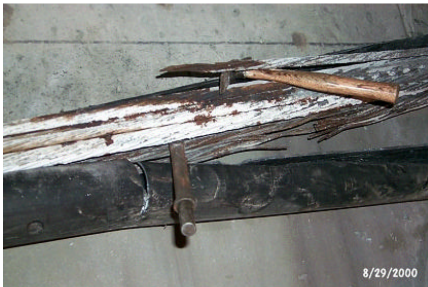
Figure 1.17 – Failure of Tendon 28-6 on the Mid-Bay Bridge
