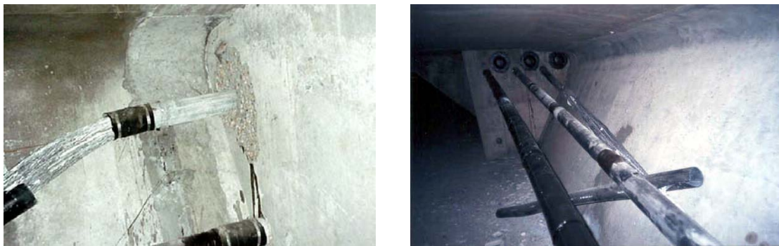
Figure 3.2 – Tendon 57-1: failure at Expansion Joint Diaphragm (left), View towards Pier Segment Diaphragm (right)
