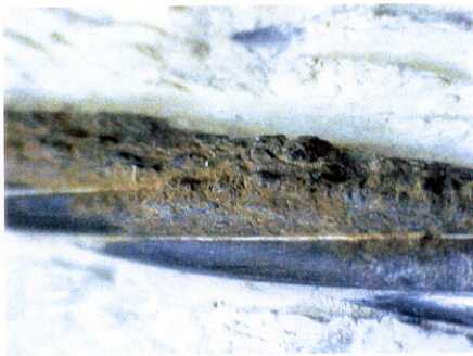
Figure 14 – Close up photograph of the corroded tendon (span 71, tendon 71-1a)
