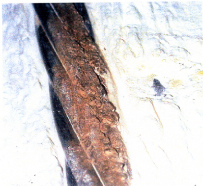
Figure 13 – Close up photograph of the corroded tendon (span 71, tendon 71-1a)
