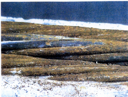
Figure 17 – Close up photograph of the corroded tendon at the 10.5 feet location (span 98, tendon 98-5c)
