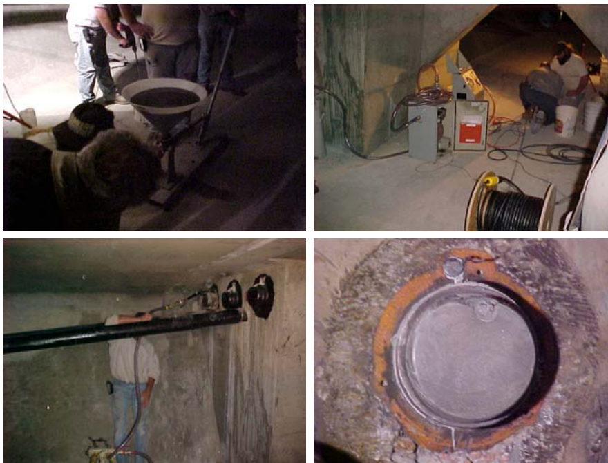
Figure 2.13 – Field trial of the vacuum injection method.
