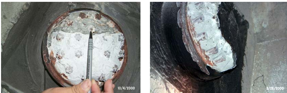
Figure 3.4 – Secondary Grout in Anchor Caps
