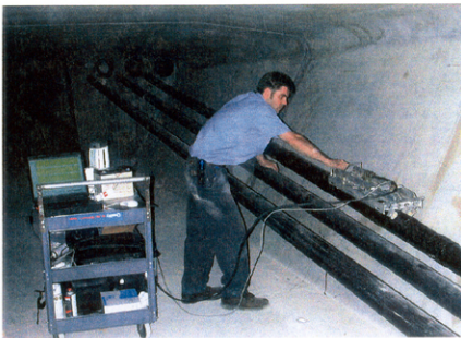
Figure 7 – Photograph of the MTTD system during a test of an external P-T tendon in the Mid Bay Bridge
