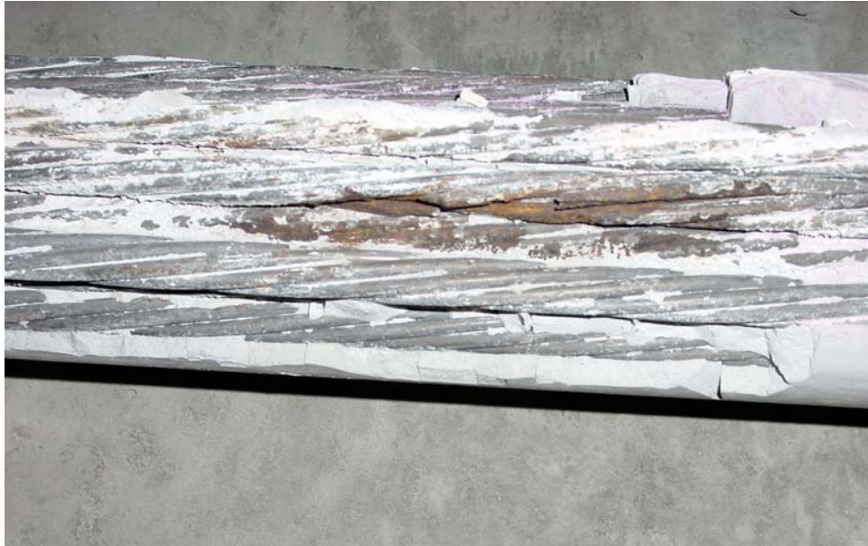
Figure 2.8 – Visual Inspection of Tendon 40-2 with corrosion in the free length of tendon.
