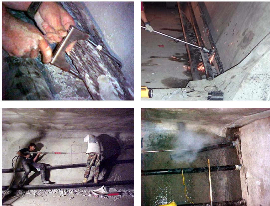
Figure 4.1 – Details of the Removal of External Tendons (Clockwise from upper left: clamping strands, cutting cable, hydro-blasting at pier segment diaphragm, and hydro-blasting operator)
