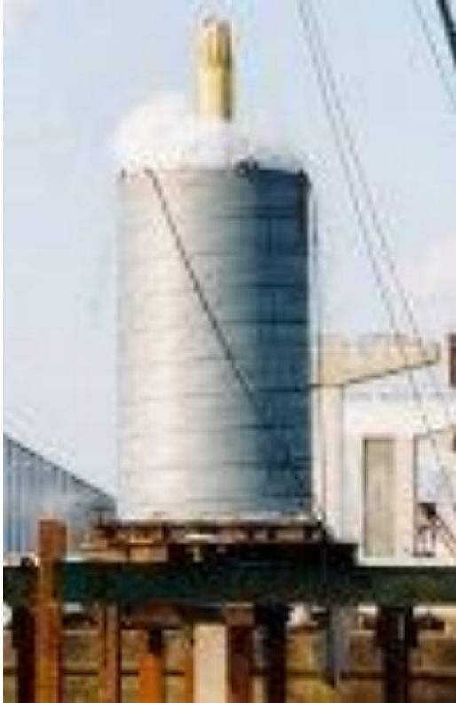
Figure 36, Axial Statnamic Load Test
