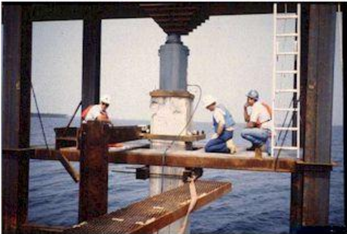
Figure 35, Static Load Test
