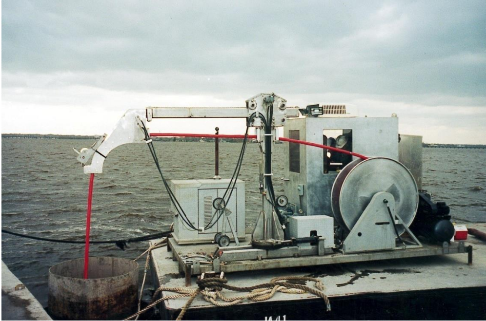
Figure 40, Shaft Inspection Device
