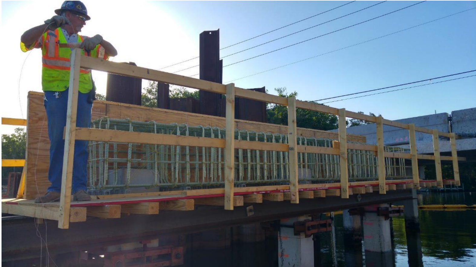
Placement of GFRP reinforcement cage at bent caps #4 and #5
