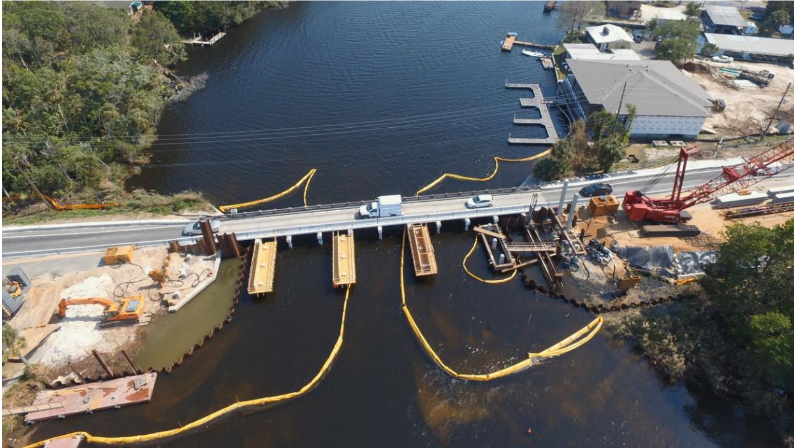
View of formwork and temporary sheet-pile installation on East side
