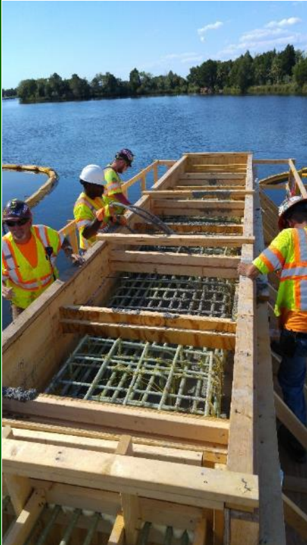
Concrete placement at bent caps #4 and #5
