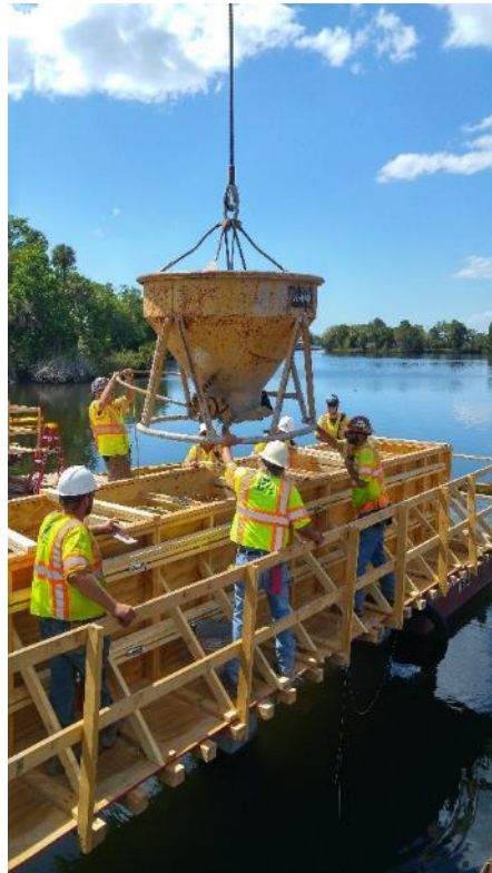
Concrete placement at bent caps #4 and #5
