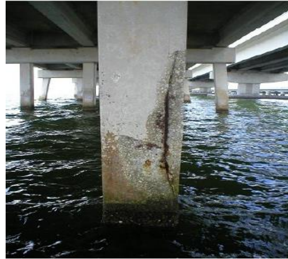
Pile Damage
