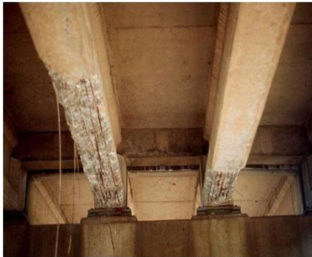
Beam Damage
