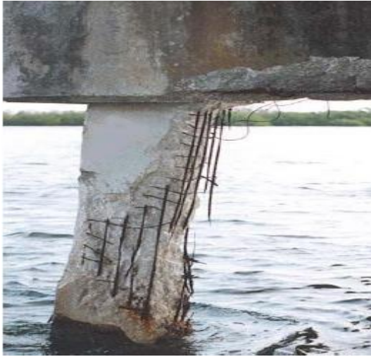
Severe Pile Damage
