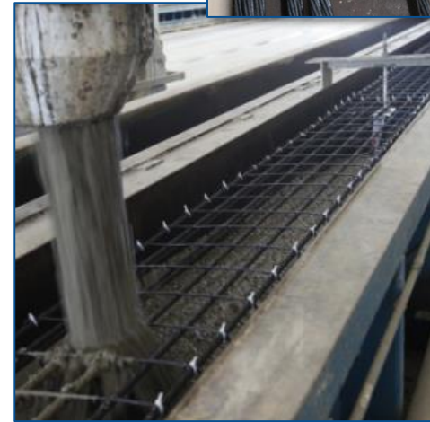
(photograph) FDOT. CFRP Pile Casting with SCC.
