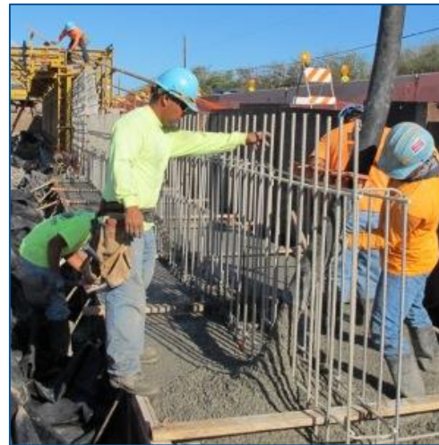
(photograph) Hughes Bros. GFRP Bars in retaining walls.
