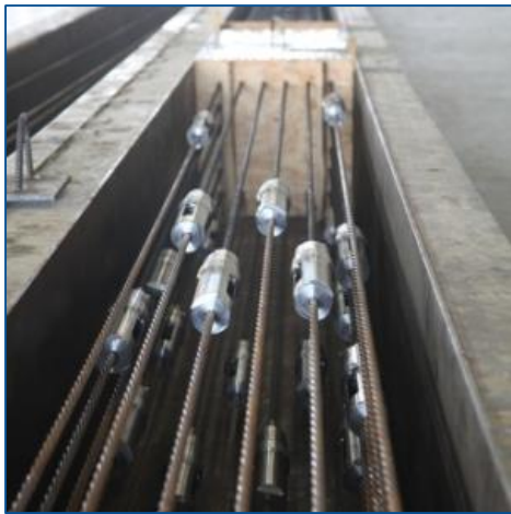
(photograph) FDOT. Coupling CFRP Strands to Steel Strands.
