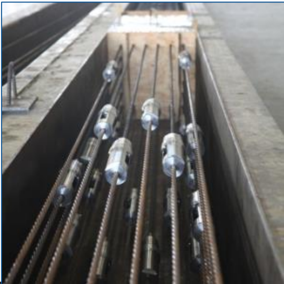
(photographs) FDOT. CFRP Strands in Piles.
