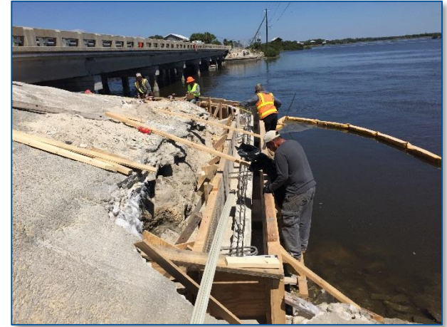
(photograph) FDOT, 2015. GFRP Bars in bulkhead cap – Cedar Key.
