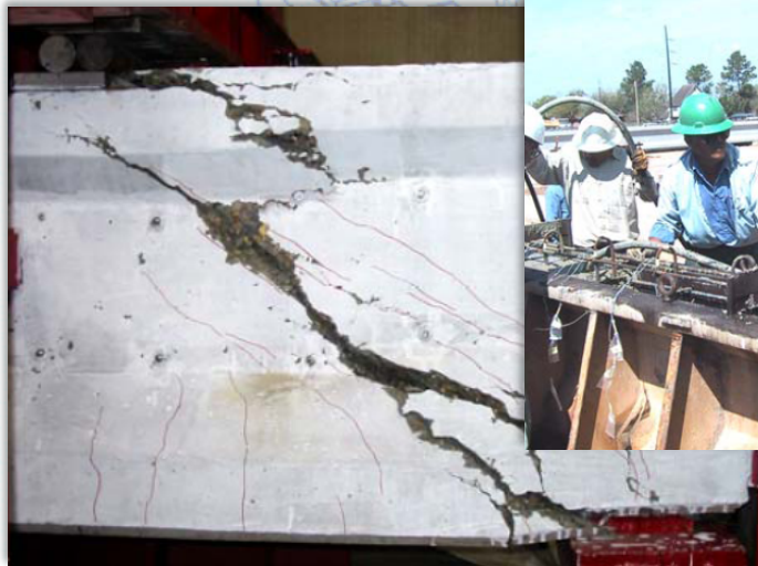
Photos courtesy of TxDOT: FHWA/TX-06/ 0-4819-1 Fiber Reinforcement in Prestressed Concrete Beams (2005)
