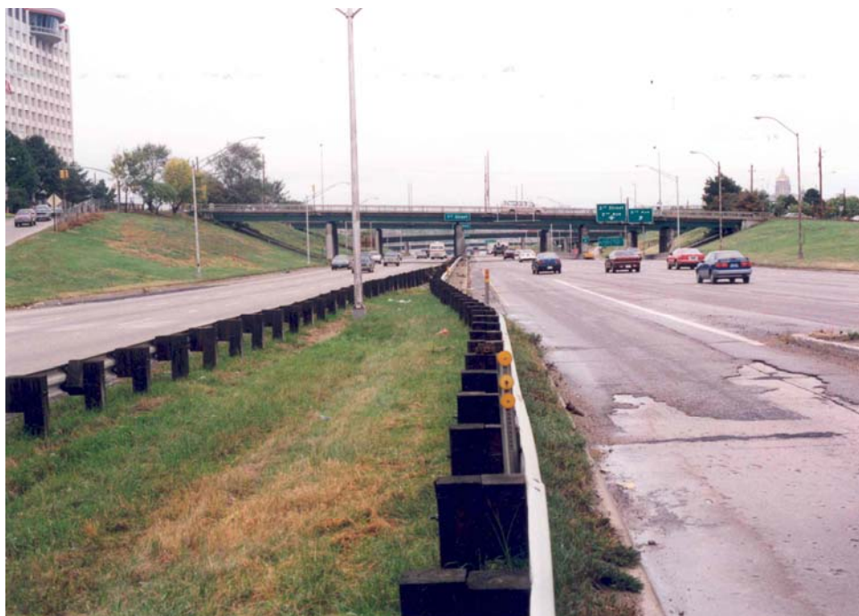
FIGURE 72 Interstate 235 before reconstruction.
