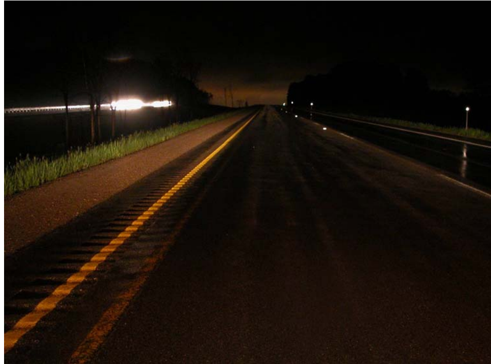
FIGURE 34 Painted edgeline rumble strips.
