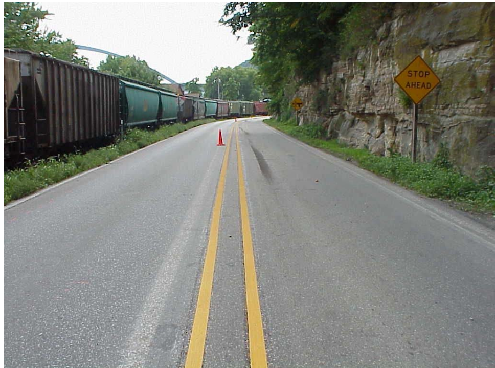
FIGURE 28 Recessed pavement markings.
