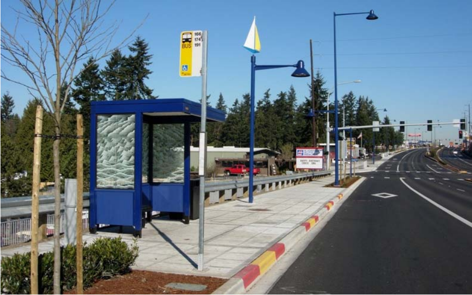
FIGURE 102 New transit stop in Des Moines.
