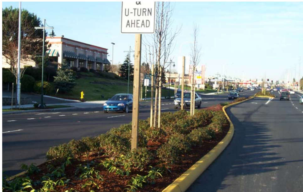
FIGURE 101 Left-turn lane and U- turn areas after reconstruction in Federal Way. A much greater level of access control was achieved.
