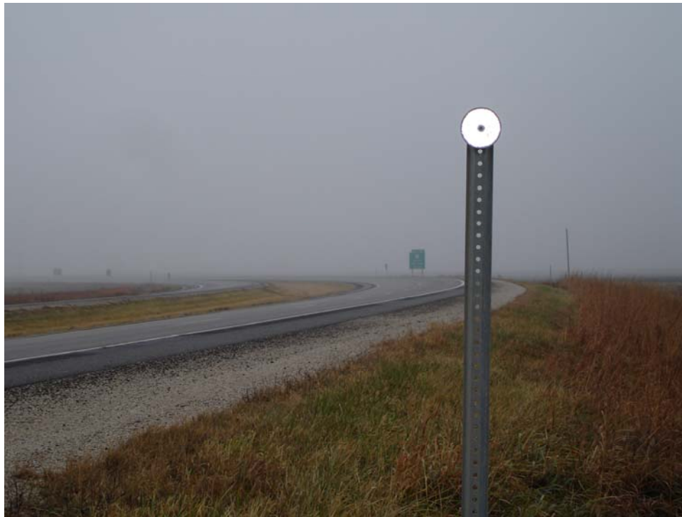
FIGURE 30 Post-mounted delineators.
