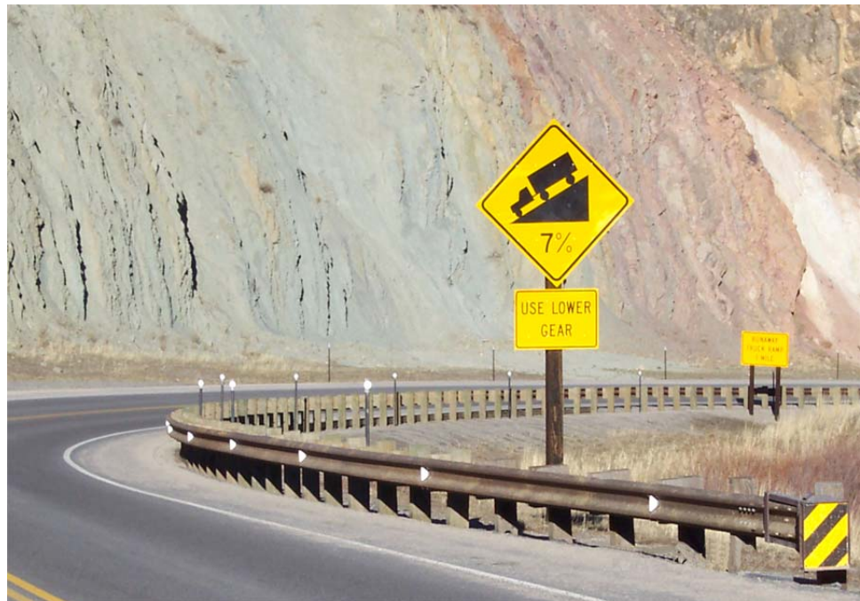
FIGURE 86 Signing for the steep grades is provided throughout the project.
