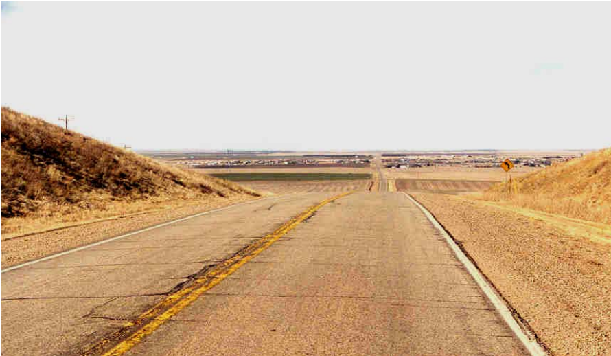
FIGURE 21 Not all locations with limited stopping sight distance are the same in terms of safety risk. In this example, the intersecting roadway in the background creates the illusion of a straight alignment and may increase the risk of run-off-road crashes.
