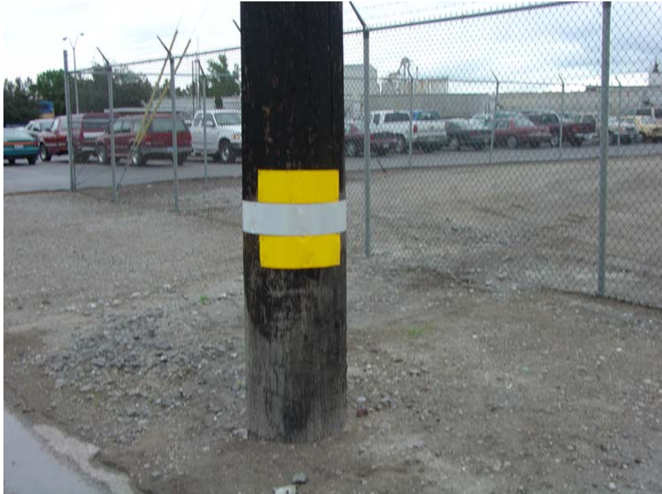
FIGURE 69 Reflective sheeting on utility poles.
