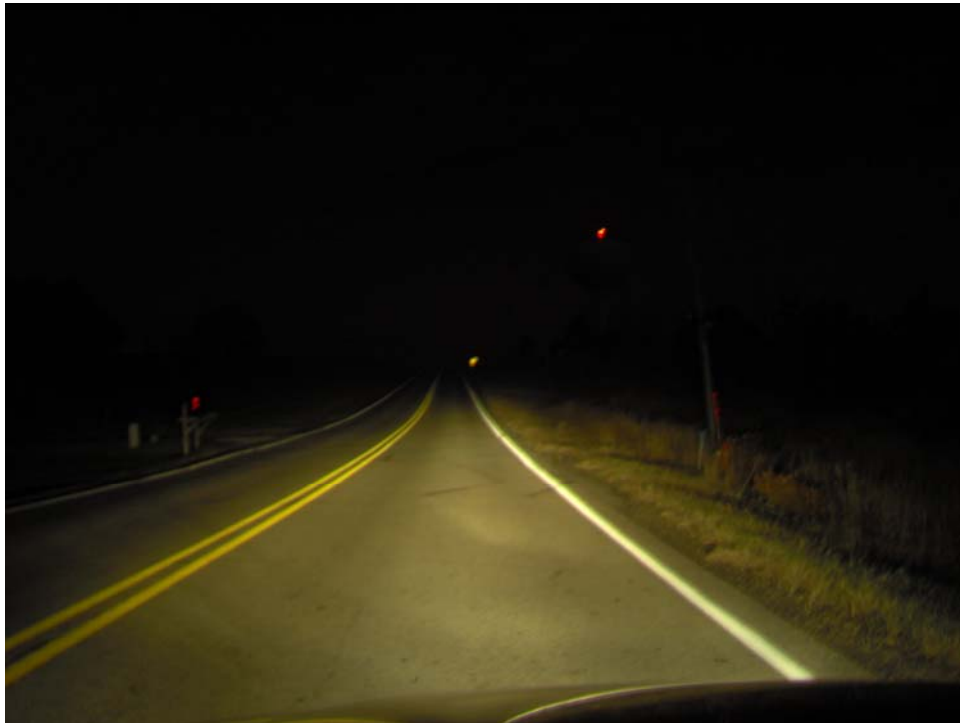
FIGURE 18 Headlight sight distance at a sag vertical curve.
