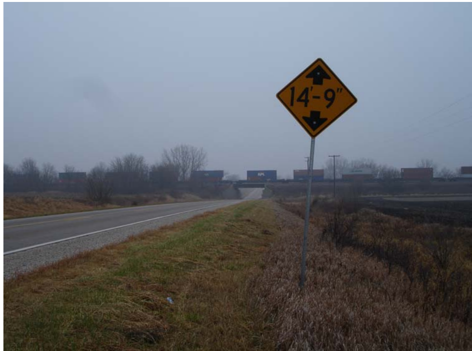
FIGURE 65 Vertical clearance signing.
