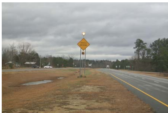
FIGURE 58 Intersection warning sign with flashers activated by vehicles entering from the side road.
