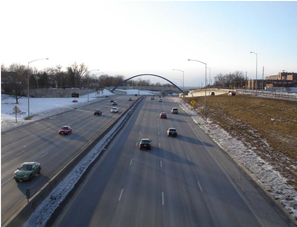
FIGURE 73 Interstate 235 after reconstruction.
