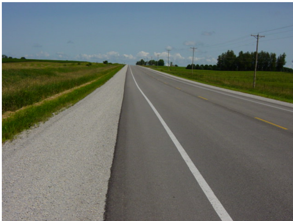
FIGURE 35 Partially paved shoulders.
