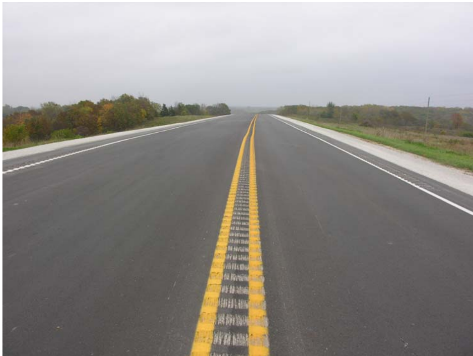
FIGURE 33 Centerline rumble strips.
