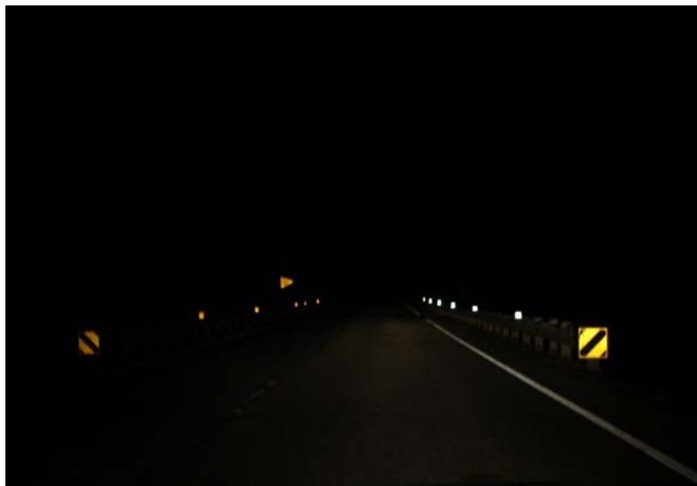
FIGURE 42 Reflector tabs on guardrail.
