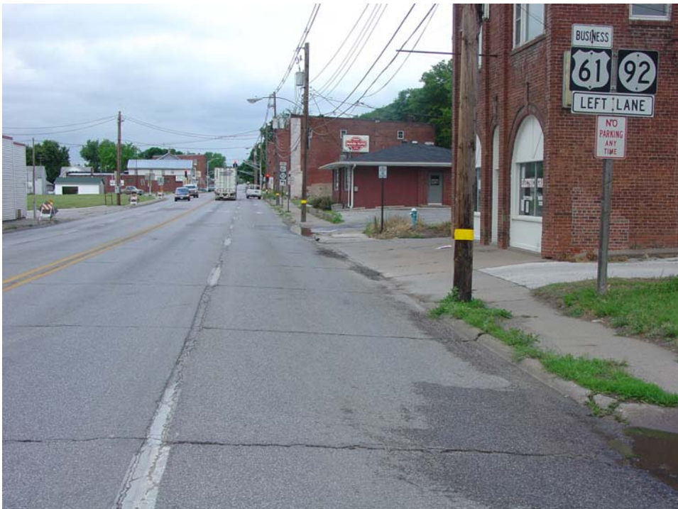
FIGURE 68 Reflective sheeting on utility poles.
