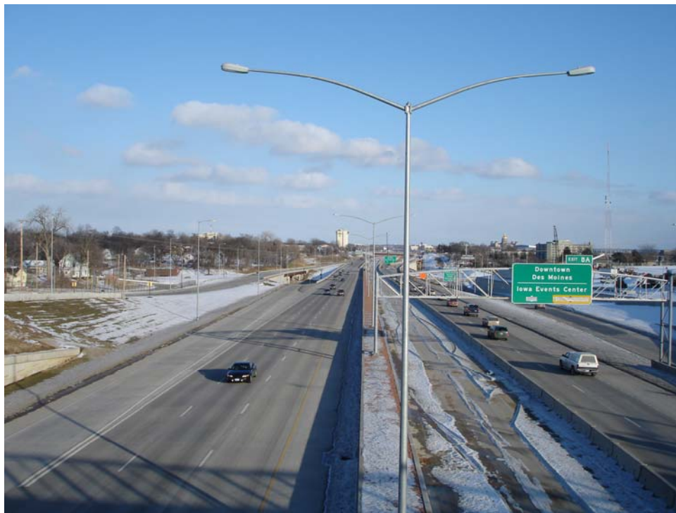
FIGURE 80 Lighting was placed down the center of the median where more cross-sectional width was available.
