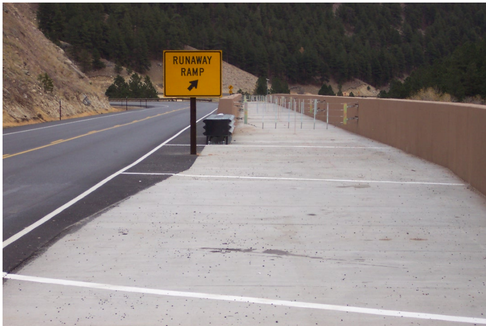
FIGURE 91 Runaway truck ramp with arrestor system.
