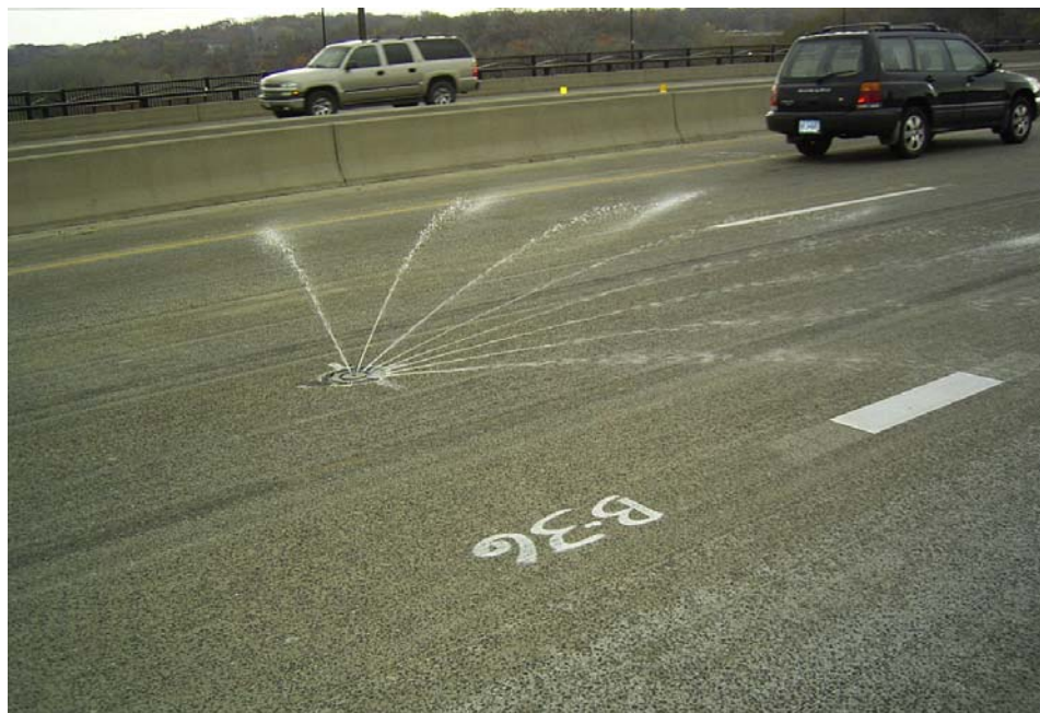
FIGURE 45 Anti-icing system on a bridge.
