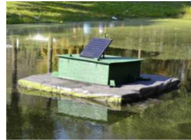
The solar panel on top of the floating media bed reactor installed in the East Palatka pond powers a pump that moves water through the filtration media and back into the pond.
