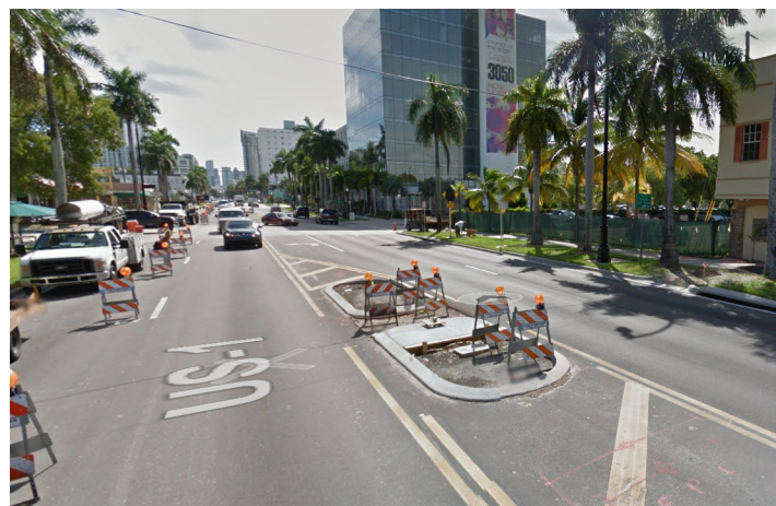
The Biscayne Boulevard corridor in Miami, specifically the intersection with NE 33rd St, was ranked the number one intersection for pedestrian crashes. Efforts to improve the safety of this location included new signage, high emphasis crosswalks, and mid-block pedestrian refuge medians. Source: Google Street View
