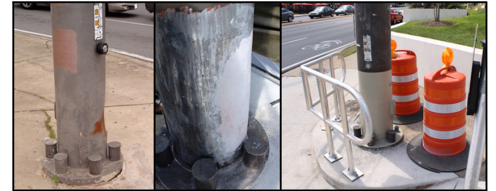
A dented utility pole in Tallahassee was chosen as a field test of the FRP pole repair system. Left: The pole was dented but still usable. Middle: After sanding, the dent is filled with epoxy. Right: After FRP application and painting, the pole is back in service without major maintenance of traffic operations.
