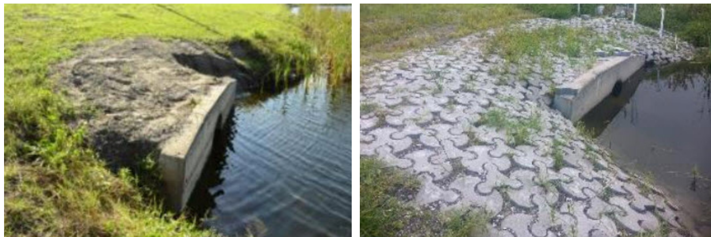
The Royal Palm Estates pond was experiencing severe erosion, as evidenced in the photograph on the left. After being graded, Tri-Lock, a concrete bank stabilization product was installed and vegetation allowed to grow in the cracks. In the months following installation, no evidence of erosion was found.
