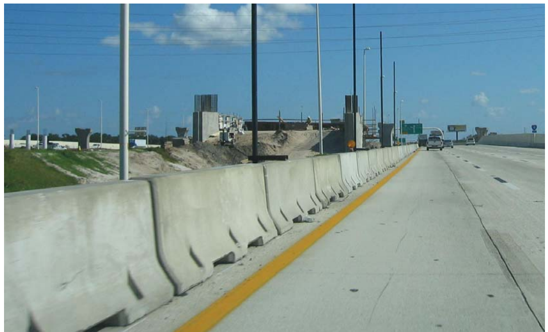
Eastbound I-4 at the CSX Railroad overpass. The contractor for the I-4 to Selman Expressway expansion project used K-barriers along the length of the five-mile project. Bolting the barriers to concrete reduces the distance barriers deflect if struck by an errant vehicle and reduces the size of the deflection zone required in work zones.
