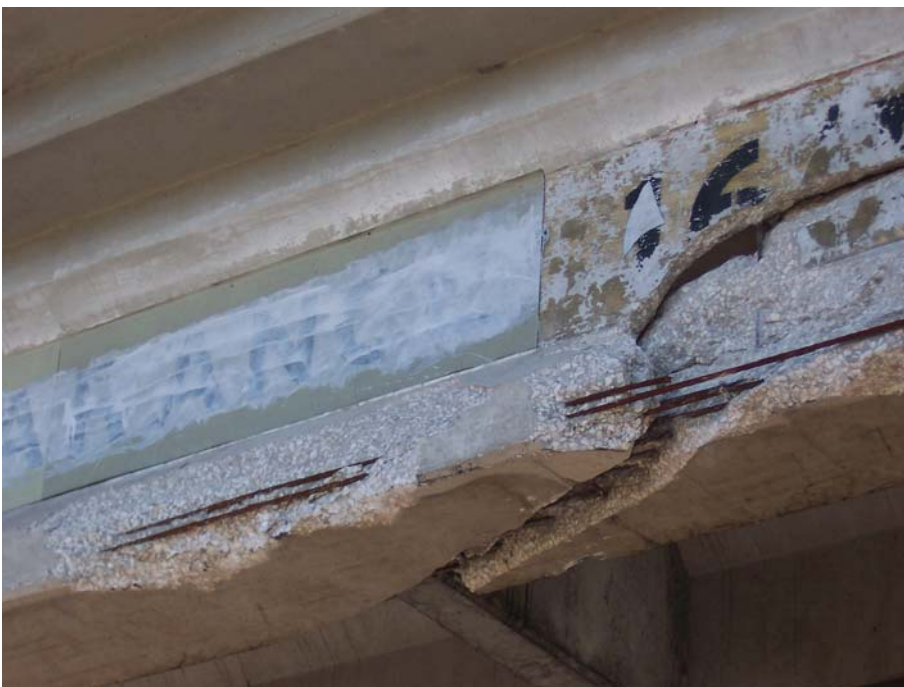
Left: Damage similar to this occurred to the Chaffee Road Bridge in Jacksonville in 2001 when it was struck by an over-height vehicle.
