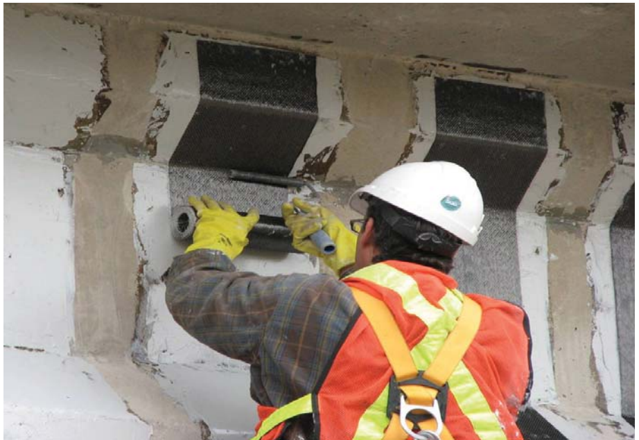
Above: A technician applies CFRP wraps to a bridge girder.
