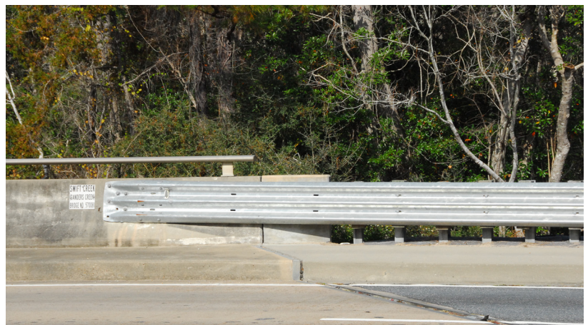
Repaving has made the ramp of the Sander's Creek bridge today nearly level with the bridge.
