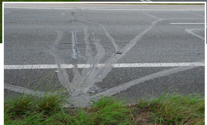
(Above and right) Inductive loop detectors on U.S. 301 between Waldo and Starke, Florida.
