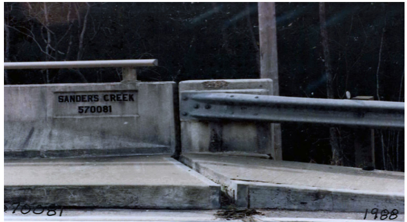
The Sander's Creek bridge 20 years ago clearly shows the ramp sloping due to soil compression.
