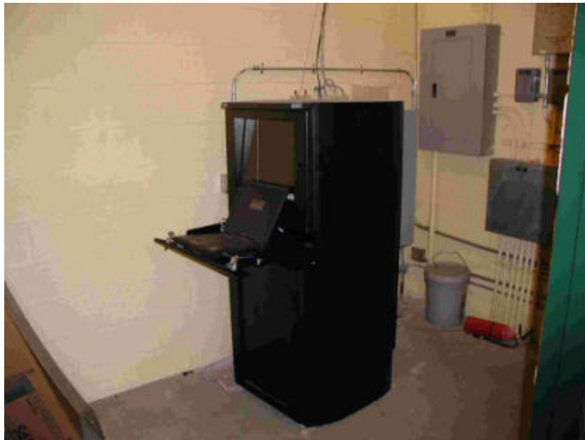
Figure 15 Rail CrossingGuard Server Installed at Cypress Creek Station
