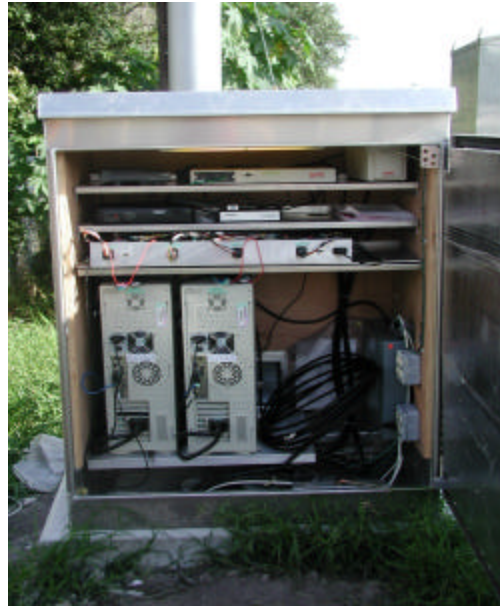
Figure 9 Rail Crossing Guard Trackage Station
