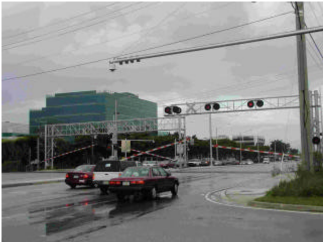
Figure 10 Signal Cameras Installed at Cypress Creek Road
