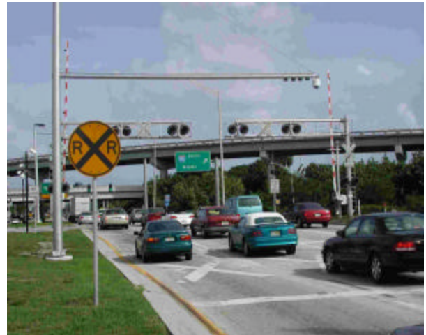
Figure 11 Signal Cameras Installed at Commercial Boulevard
