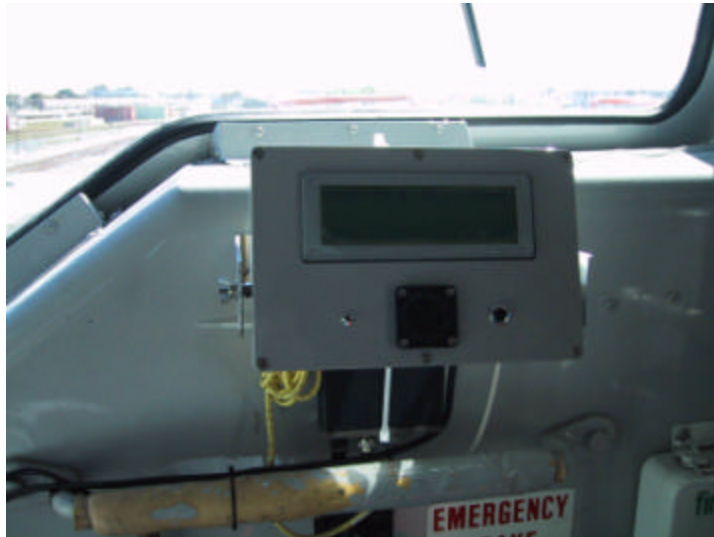
Figure 12 MMIT Installed in Locomotive
