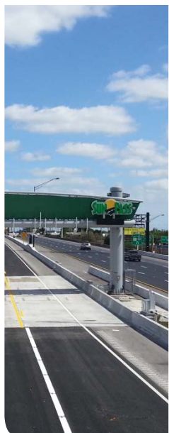
4208093: I-595/SR-862/P3/CEI From East of I-75 to West of I-95
