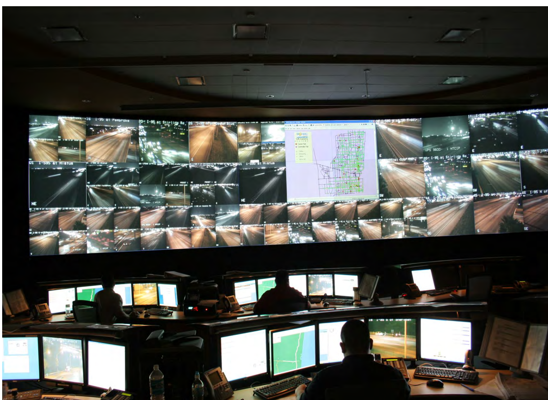
Regional Transportation Management Center
